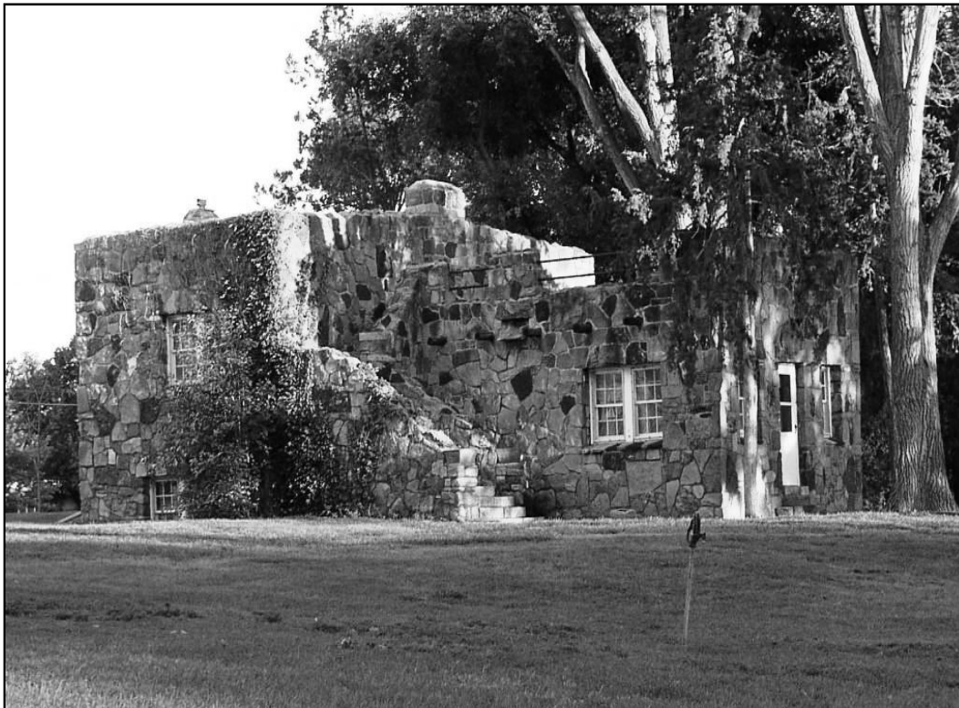
Figure 20: The caretaker's residence at Willow Creek Park in Lamar, Prowers County, shows the influence of both rustic park architecture and the Pueblo Revival style. Photo: Deon Wolfenbarger, June 2004.
