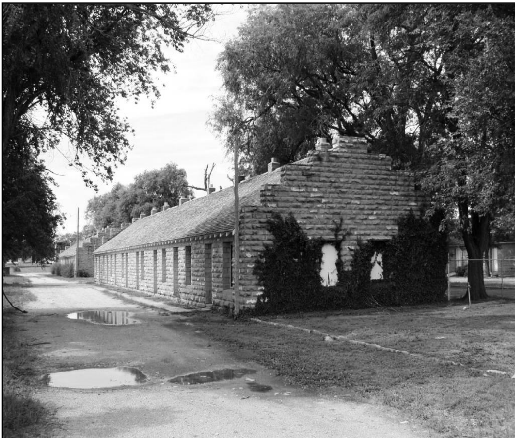
Figure 12: Five buildings were constructed in separate phases for the Prowers County Welfare Housing project. The buildings included housing, a laundry/restroom facility, and commodities distribution offices. Photo: Deon Wolfenbarger, June 2004.
