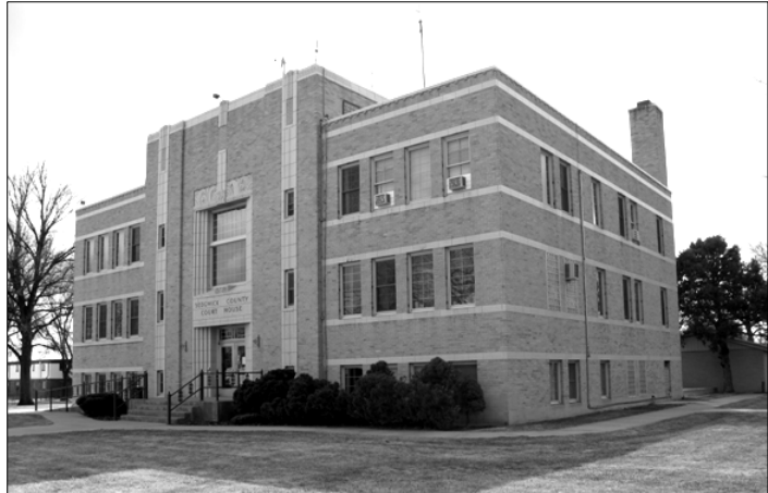
Figure 21: The Sedgwick County Courthouse exhibits the vertical orientation and simple ornamentation representative of WPA Art Deco.
