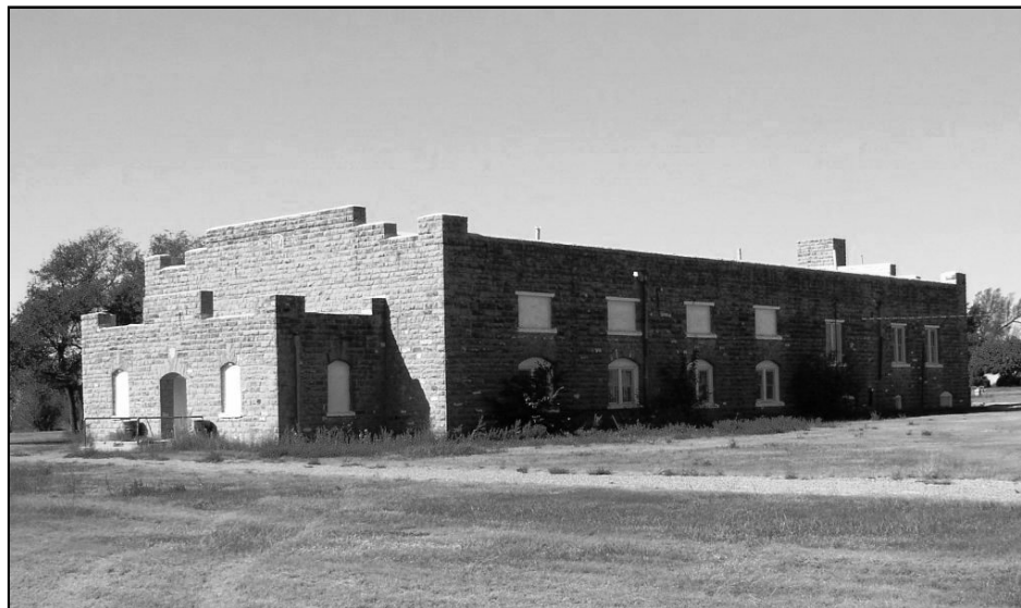
Figure 17: Top - Holly Gymnasium in Prowers County, built of Niobrara stone, a chalk-like substance soft enough to quarry with hand-saws, but which hardened upon exposure.
