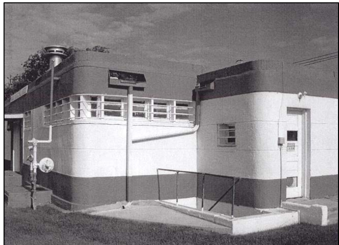
Figure 22: The Bath House at the Hugo Swimming Pool features the rounded corners and horizontal orientation of WPA Moderne.
