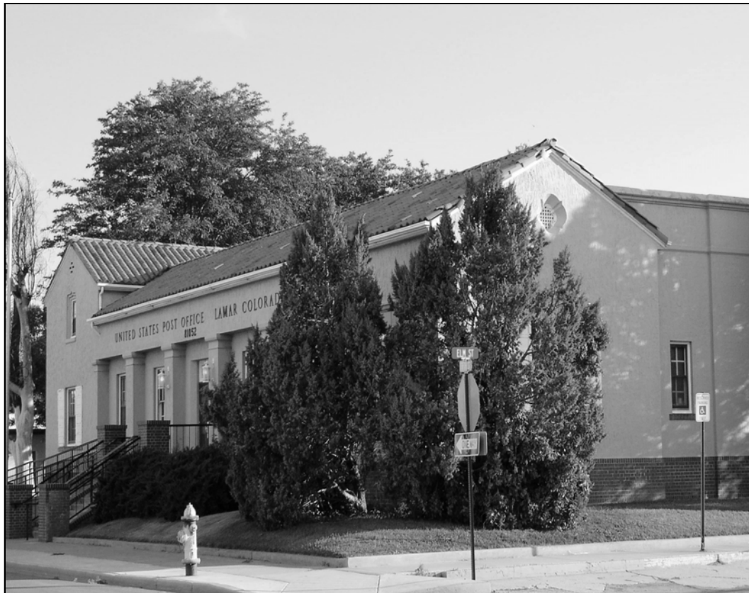
Figure 9: According to the authors of the 1939 review of PWA architecture, the Lamar Post Office exhibits several of the hallmarks of a federal project from region 5: use of a regional style, thick walls, reinforced concrete construction covered with stucco, and small windows to reduce heat loss. Photo: Deon Wolfenbarger, June 2004.
