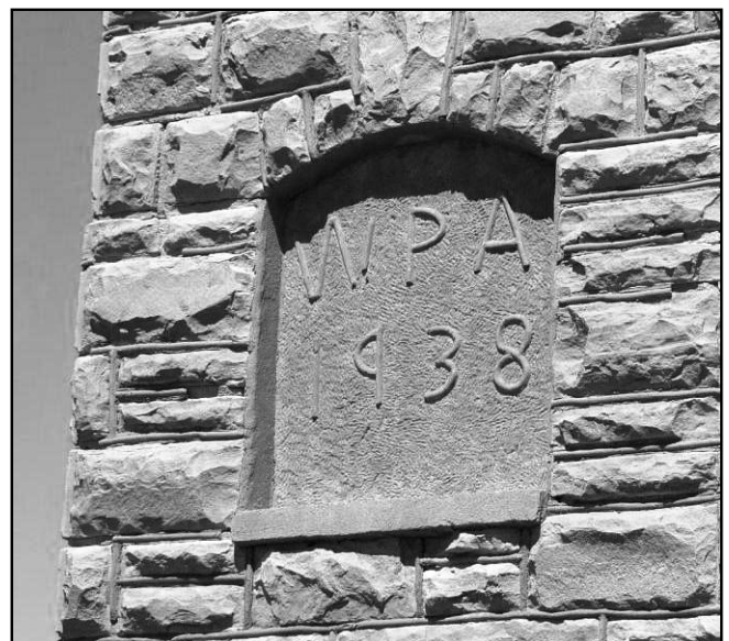
Figure 14: Raised beaded mortar lettering on a concrete stippled background give a folk art quality to the Konantz School in Baca County. Photo: Deon Wolfenbarger, October 2004.
