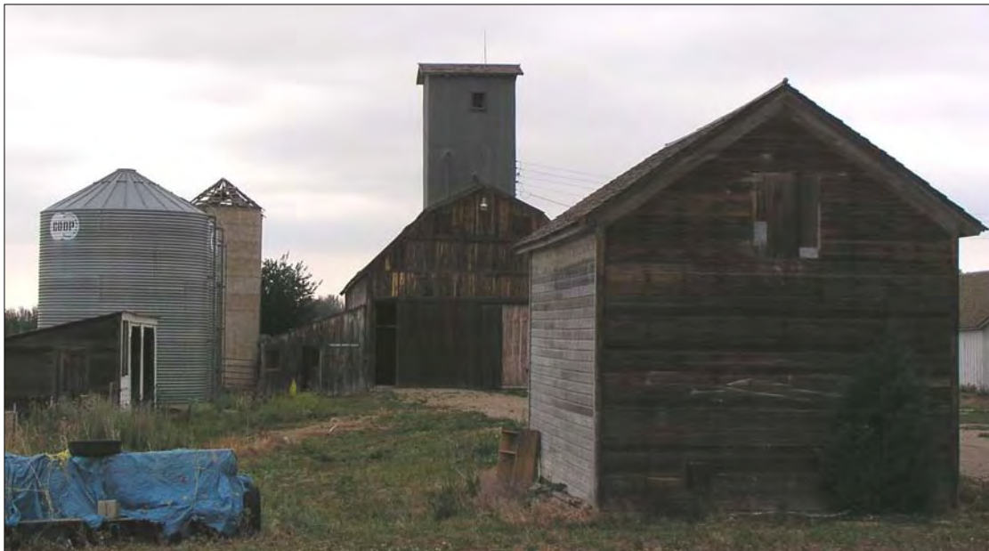
An evolution of grain storage structures can be found at 7016 N. 73 rd Street, including a granary, concrete stave silo, and prefabricated metal bins.
