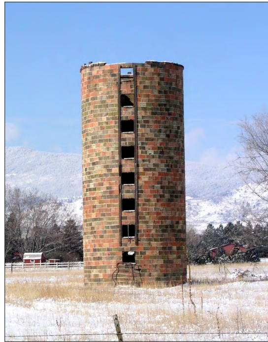
Hollow glazed clay tile silo.
