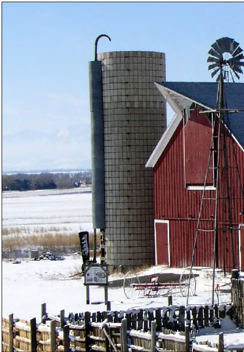
Concrete stave silo adjacent to barn at Lohr/McIntosh Farm.
