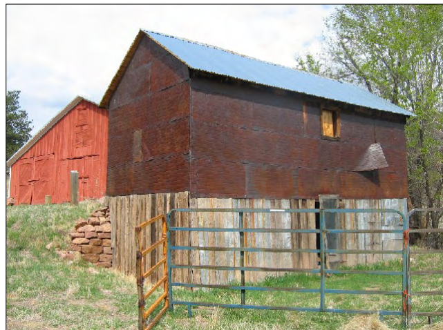
Hall Ranch bank barn.
