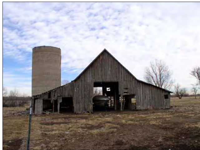
The Henning Farm barn—a Midwest three-portal barn formed by shed additions to the sides.
