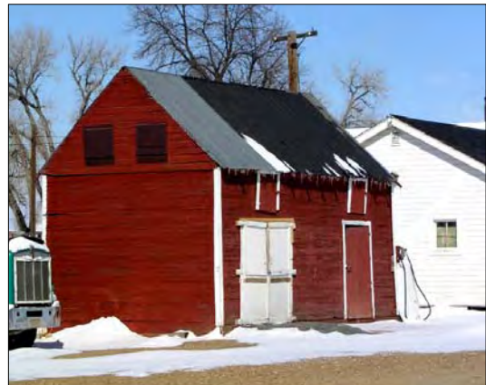
Stacked plank granary on Ute Road
