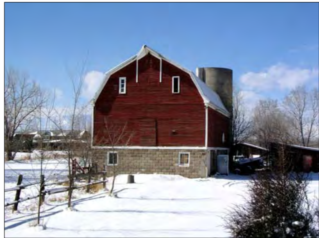
Dairy barn in Hygiene with concrete block construction on the lower portion for ease in cleaning.
