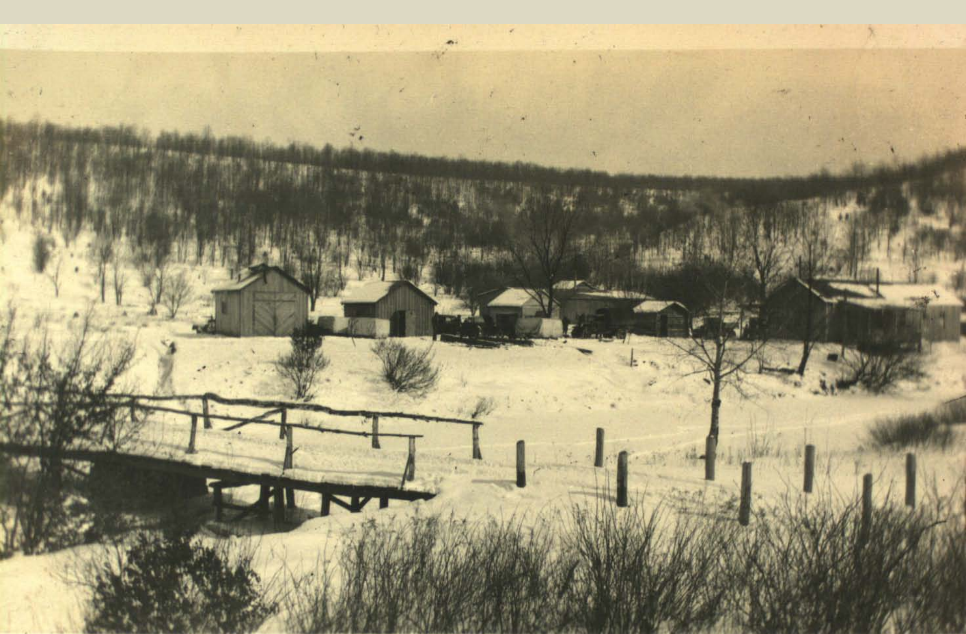
The men also built the bridge over Spring Creek into camp.
