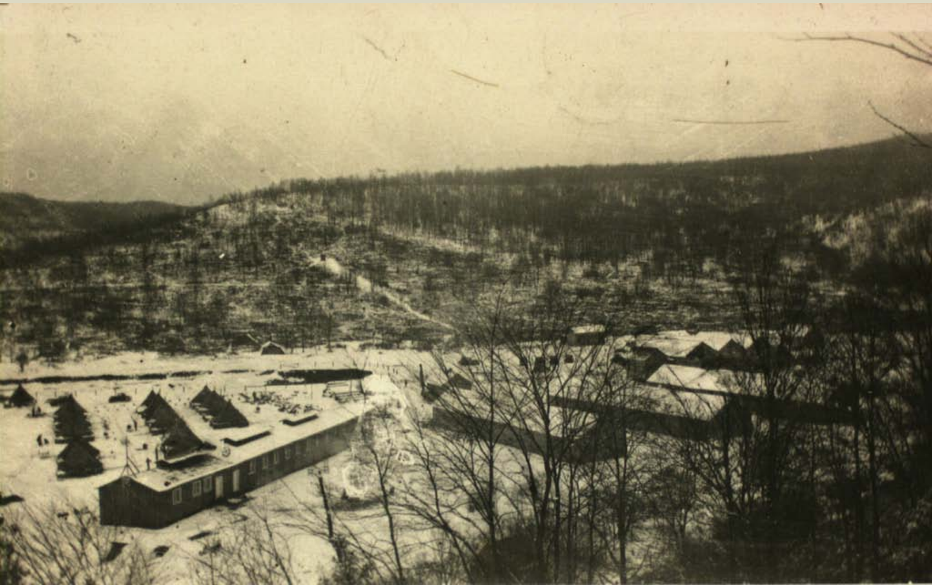
Following completion of the Mess Hall, the men constructed 3 barracks along Sp
