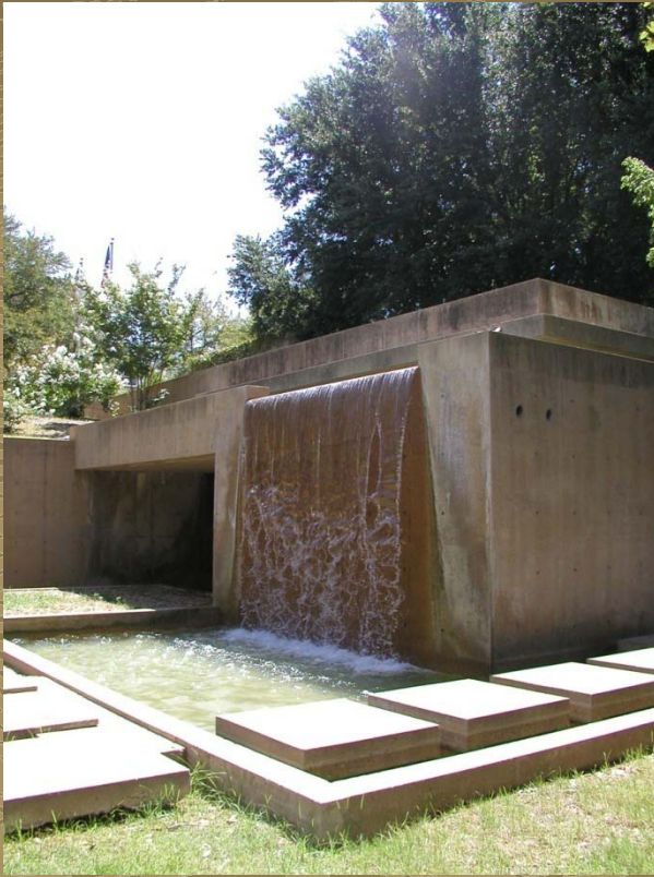
Heritage Park Plaza Fort Worth, Texas Designed by Lawrence Halprin Photo courtesy of Historic Fort Worth, Inc.
