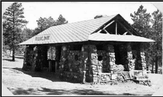
Fillius Park Shelter (1918).
