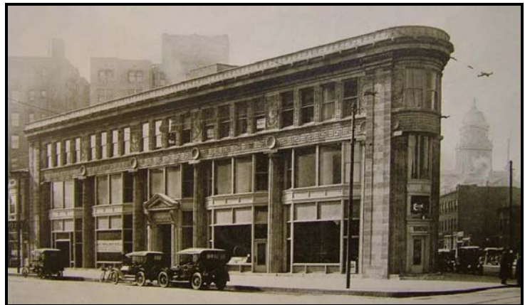
Flat Iron Building (1913).
