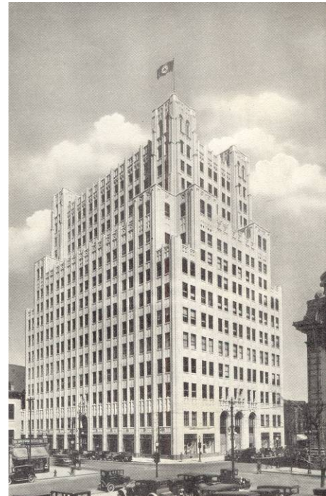
Bowman designed Telephone Building in Denver
