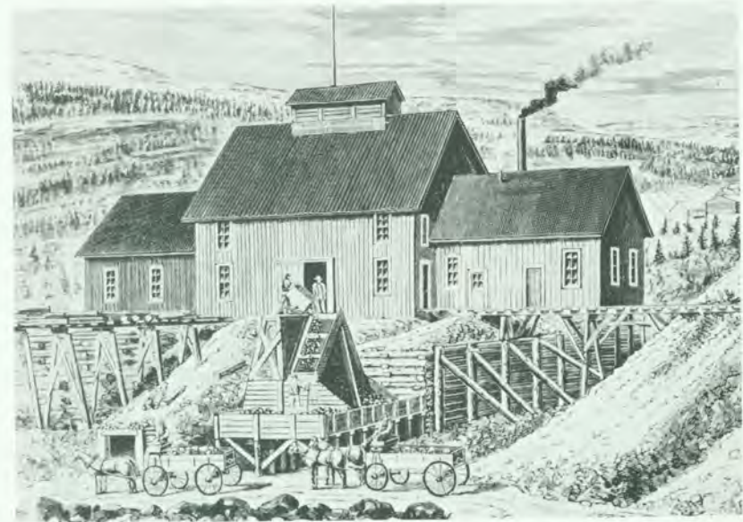
The main shaft of the Little Chief Mine.
