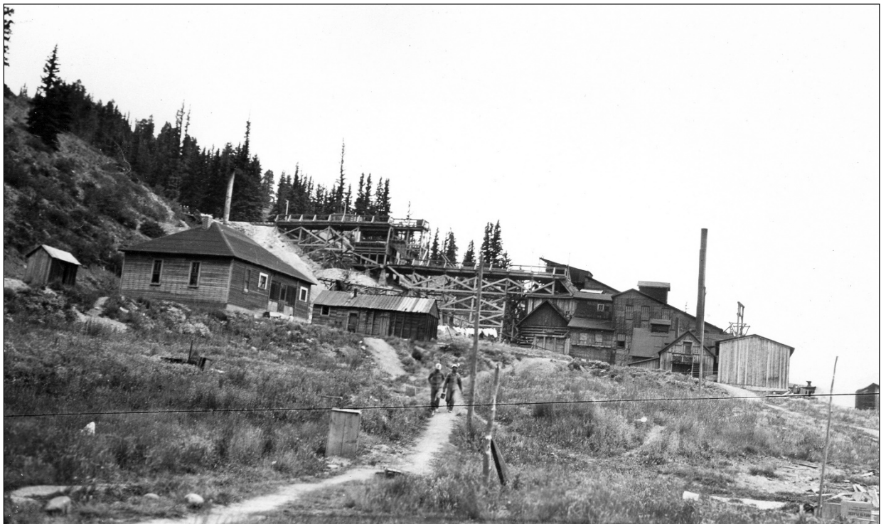
H1. View of the north side of the mill and trestle taken in 1926 by E.E. Burchard. USGS Photo 1324
