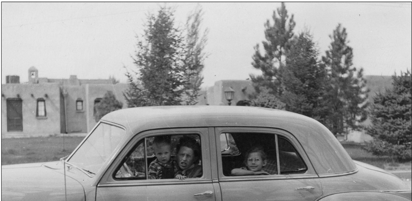
Figure 4. View north of the Coronado Lodge from Aqua Avenue, showing the south wall (rear) of Resource 4. SOURCE: John Ercul photograph collection, Pueblo, Colorado, ca. 1954.
