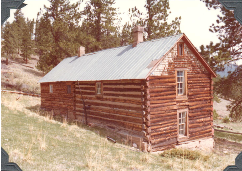
Photo HP1. Main House, view to the north showing south and west façades, 1979 (Dargan 1979).
