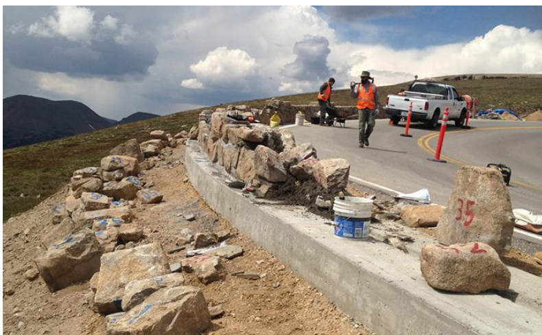
Rebuilding rock wall, Trail Ridge Road
