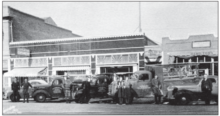
In 1941, IREA moved into its first Littleton office, located at 2449 W. Main Street. The building and fleet are shown here in 1942. Photo: Courtesy of IREA, from the Summer 1975 Watts & Volts .
