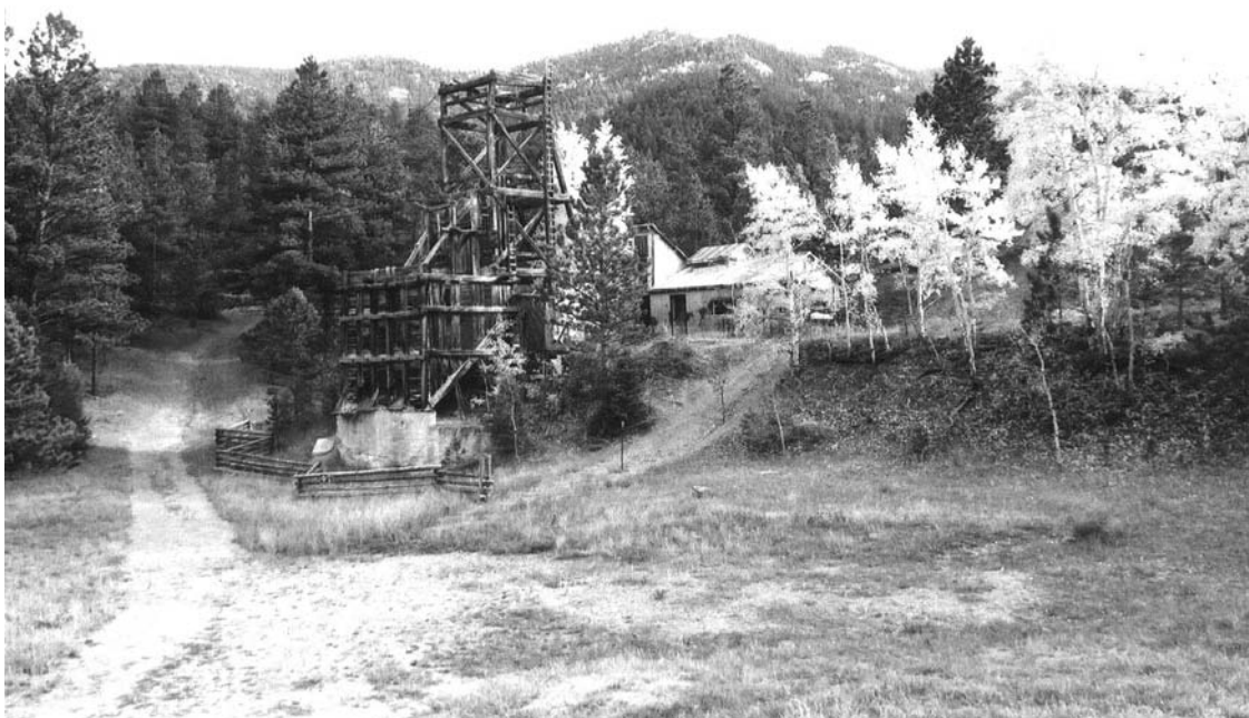
Figure E 4.9.4. In 1940, Harry M. Williamson & Son their small fluorspar empire when they leased the Blue Jay, Emmitt, and Argo mines and operated the properties together. The firm installed similar surface plants at all three mines, and the one at the Blue Jay is currently the best-preserved. Source: Author.
