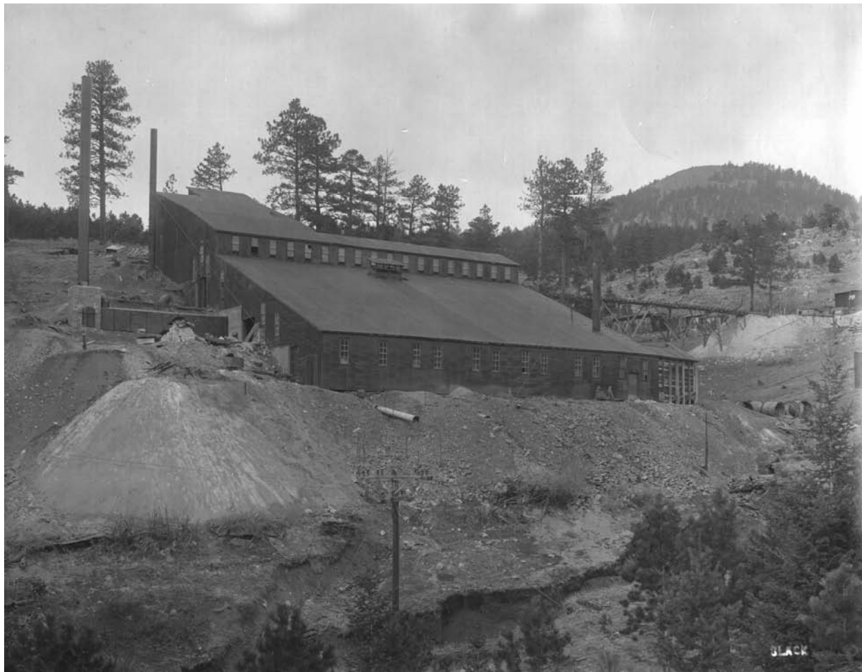
Figure E 4.8.4. The United States Gold Corporation tinkered with the massive and costly Livingston Mill for around ten years but never ran it at capacity. Intermittent operations, changes in ownership, and lack of production between 1907 and 1918 roused suspicions that the mill was a fraud. Source: Boulder Carnegie Library, 219-5-14.
