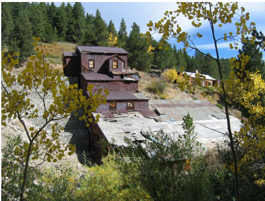
Figure E 4.3.4. Today's Cardinal Mill, formerly known as the Boulder County and the Midget, has changed little since it was built during the 1890s. The Boulder County Tunnel is left and out view. Source: Carol Beam.
