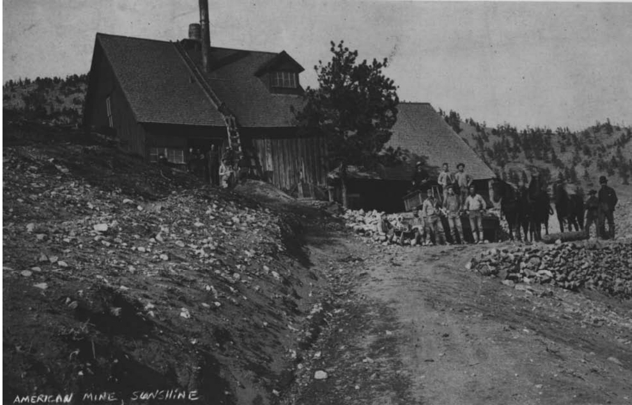
Figure E 4.7.3. New York City capitalist Hiram Hitchcock purchased the American Mine in 1876, invested in a substantial steam plant, and sank the shaft deeper. Hitchcock was amply rewarded for his expense, and the American became one of Sunshine's most important mines. The structure at left enclosed the shaft and hoisting system, and the shed at right was an ore sorting house. Source: Boulder Carnegie Library, 219-1-9.
