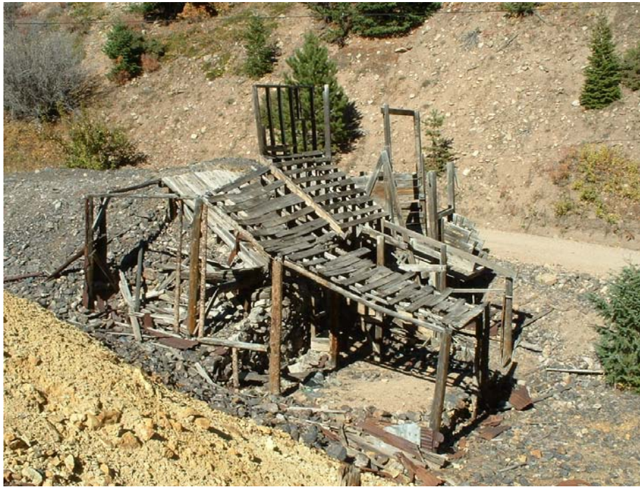
Figure E 4.2.6. In 1935, R.W. Graham built a screening station at the White Raven Mine to process waste rock. Today, only the skeleton remains. Source: Author.
