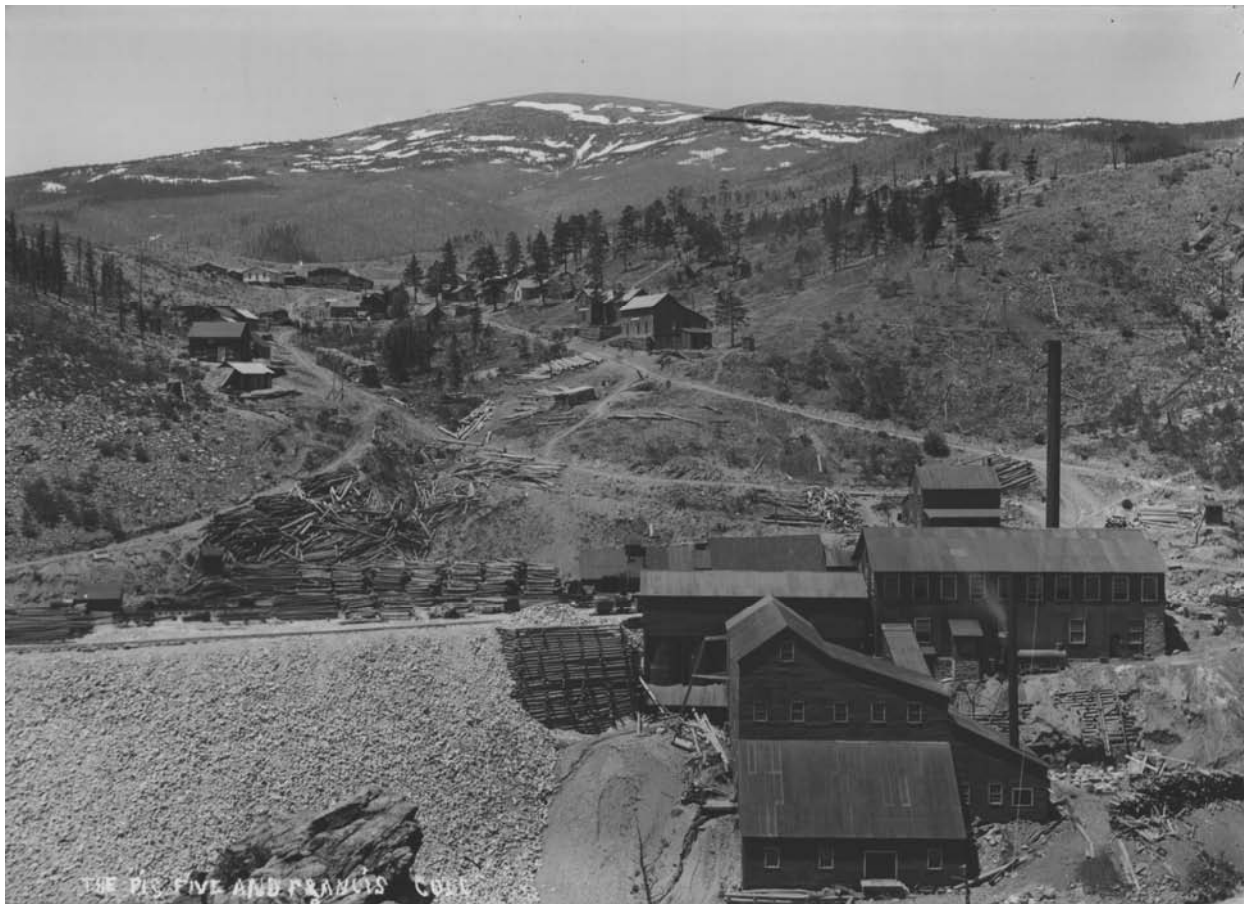
Figure E 4.2.4. The Big Five Mine, formerly the Dew Drop, was the most important operation in the Ward Mining District during the late 1890s. The Big Five Mill is at lower right, a powerhouse stands immediately above, and the stacks of cordwood stand adjacent to the Adit Tunnel. Miners employed at the Big Five and surrounding operations lived in Camp Frances, a portion of which is visible at upper left. A spur track for the Colorado & Northwestern Railroad extends right. Source: Boulder Carnegie Library, 219-3-5.
