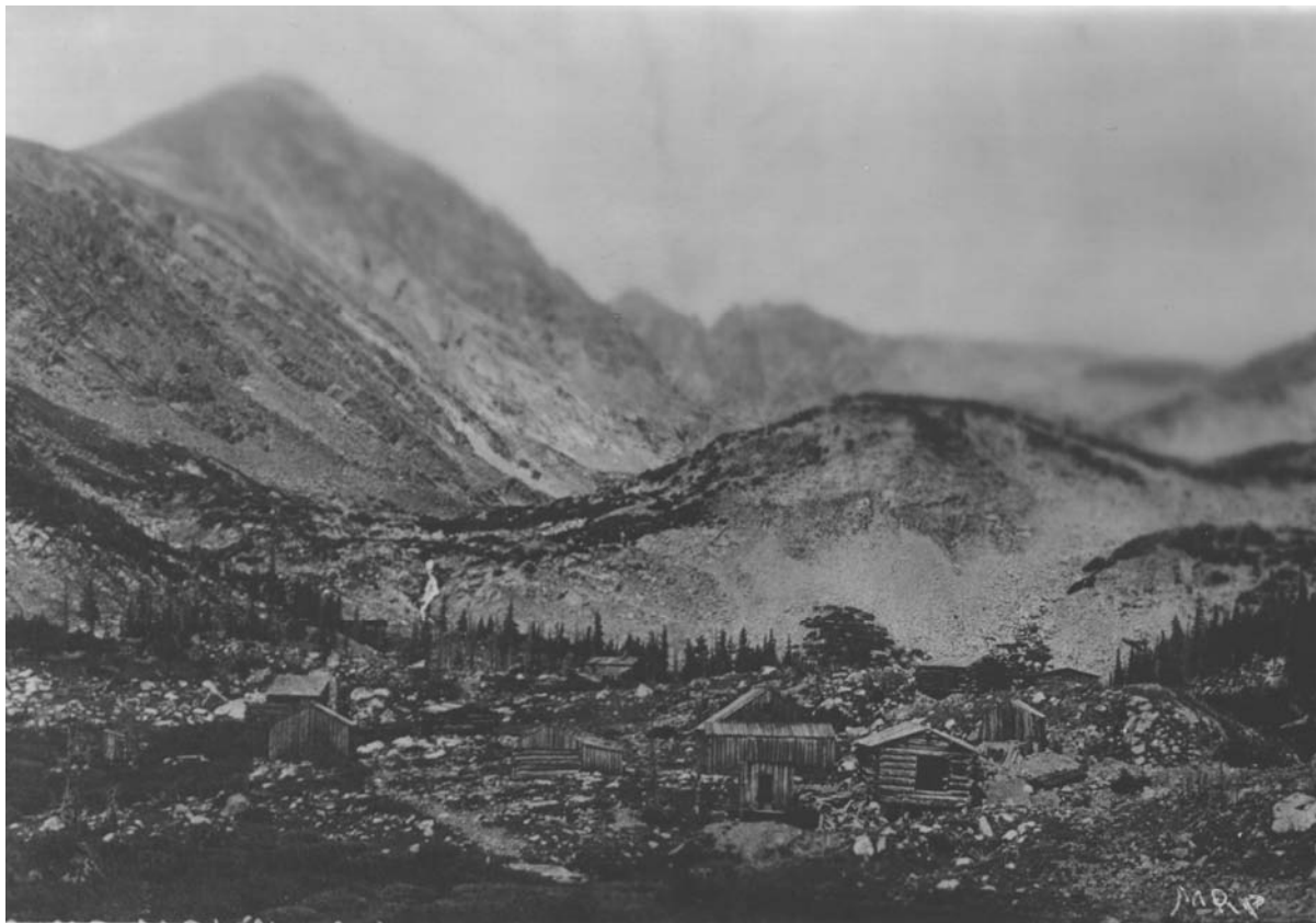
Figure E 4.4.2. Camp Albion experienced several incarnations and consisted of little more than a few prospectors' cabins, several company boardinghouses, and the Albion and Century mines, one of which is at lower center. Albion was one of the county's highest and most remote settlements. Source: Boulder Carnegie Library, 213-1-3.
