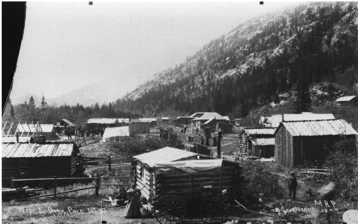
Figure E 4.5.2. Eldora exploded with activity in 1898 and 1899, and the town's boom was based on speculation instead of a proven mining industry. In this westward view, some buildings at left are still under construction. Source: Boulder Carnegie Library, 213-1-12.
