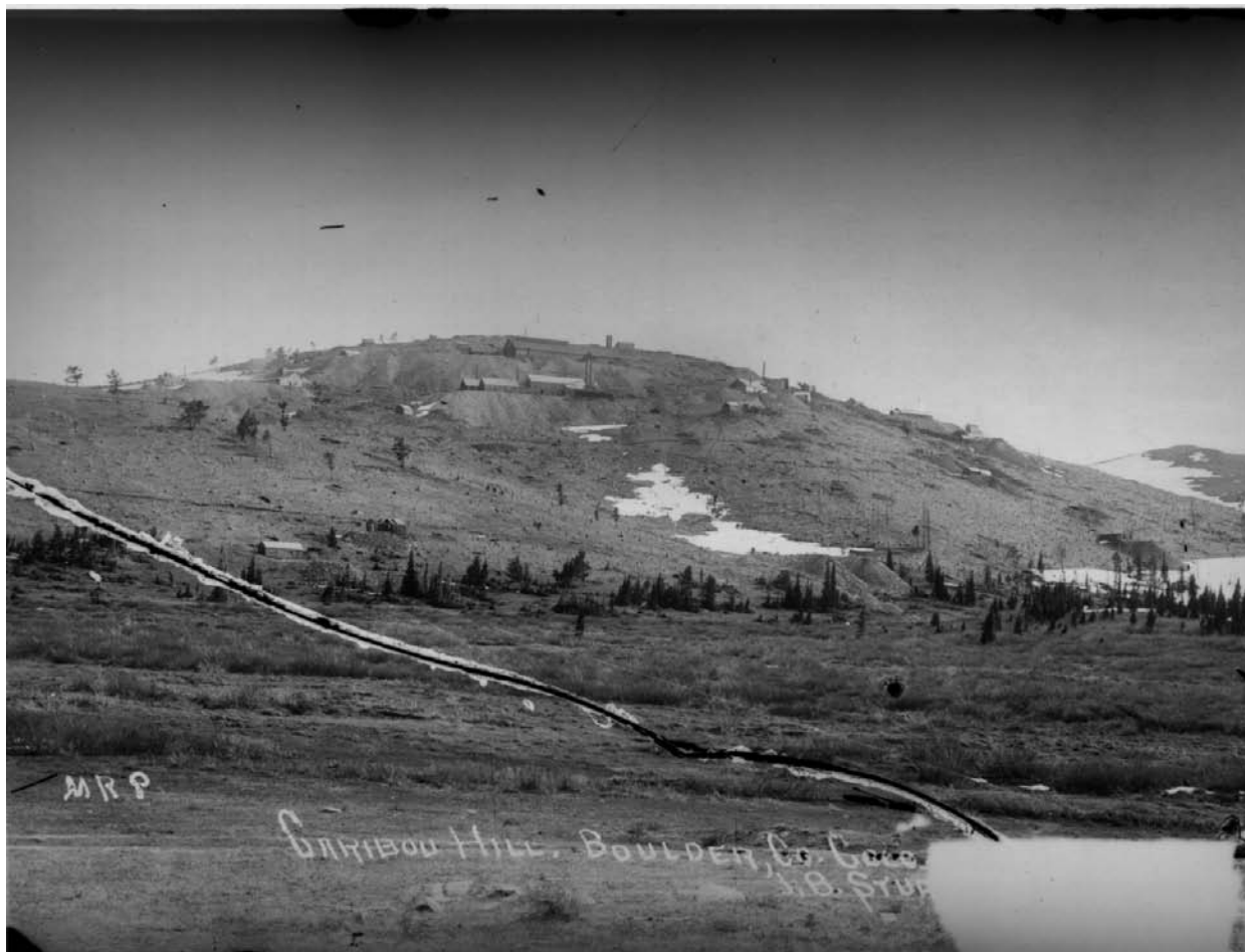
Figure E 4.3.2. Caribou Hill was the economic and industrial center of the Grand Island Mining District as it existed around 1880. The long, dark shaft house immediately below the hilltop belonged to the Caribou Mine, and the waste rock dumps at the hill base right of center mark the Seven-Thirty Tunnel. The town of Caribou is left and out of view. Source: Boulder Carnegie Library, 219-2-9.
