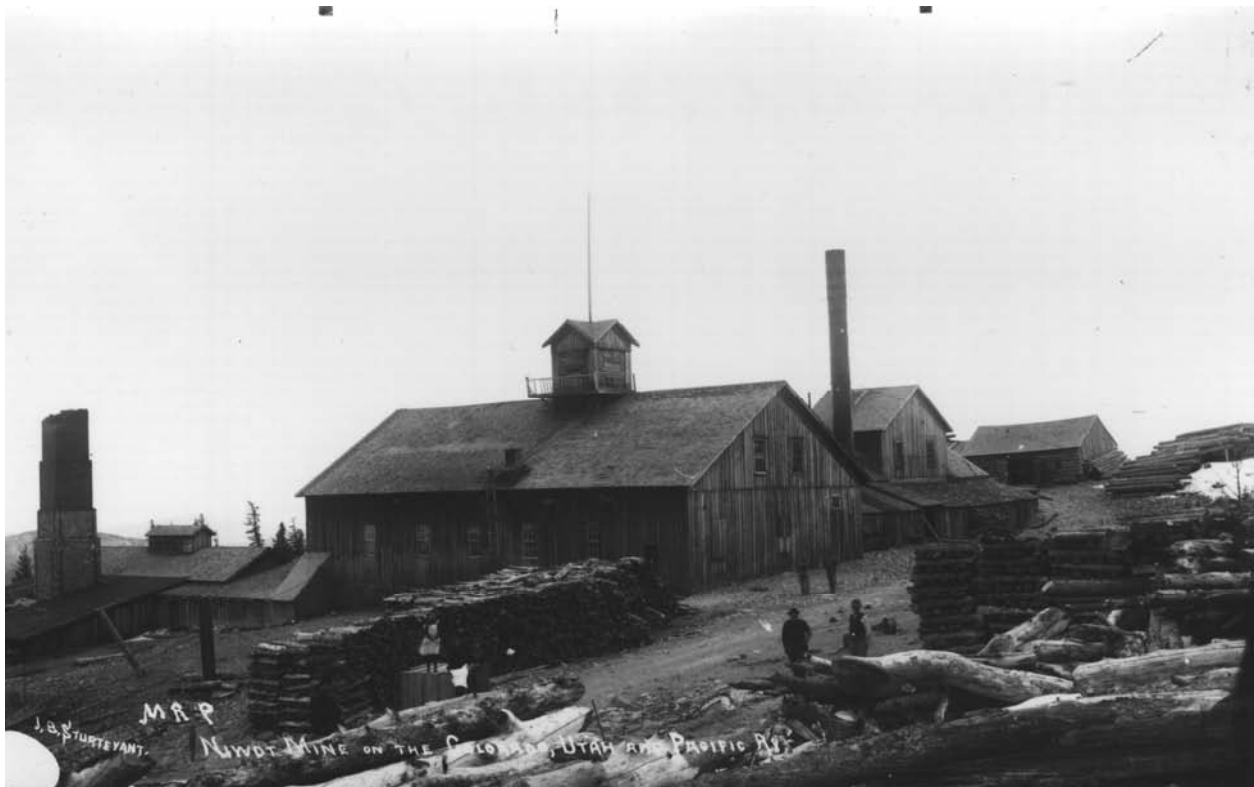
Figure E 4.2.2. The Niwot Mine was one of Ward's oldest and most important operations during the late 1870s boom. The shaft house, center, may be the original structure constructed in 1865 or 1866, and the mill, right, was crucial for the mine's success. By the late 1890s, when Rocky Mountain Joe Sturtevant took this photograph, the mill was idle and its furnace chimney in decay. Source: Boulder Carnegie Library, 219-6-24d.
