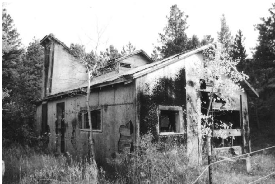
Figure E 5.2.39. After shaft houses were outlawed during the 1910s, mining companies erected hoist houses to enclose critical facilities. The Blue Jay Mine's hoist house, near Jamestown, is a typical example. The left roofline features an angled cupola for the hoist cable, which ascended to a headframe left and out of view. Source: Author.
