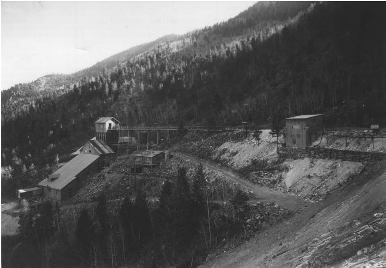
Figure E 4.6.6. Around 1934, Slide Mines built a new mill at the mouth of the Corning Tunnel. The operation was one of Gold Hill's most profitable and a significant employer, both of which were important in the climate of the Great Depression. The tunnel is right and out of view. Source: Boulder Carnegie Library, 219-8-9b.
