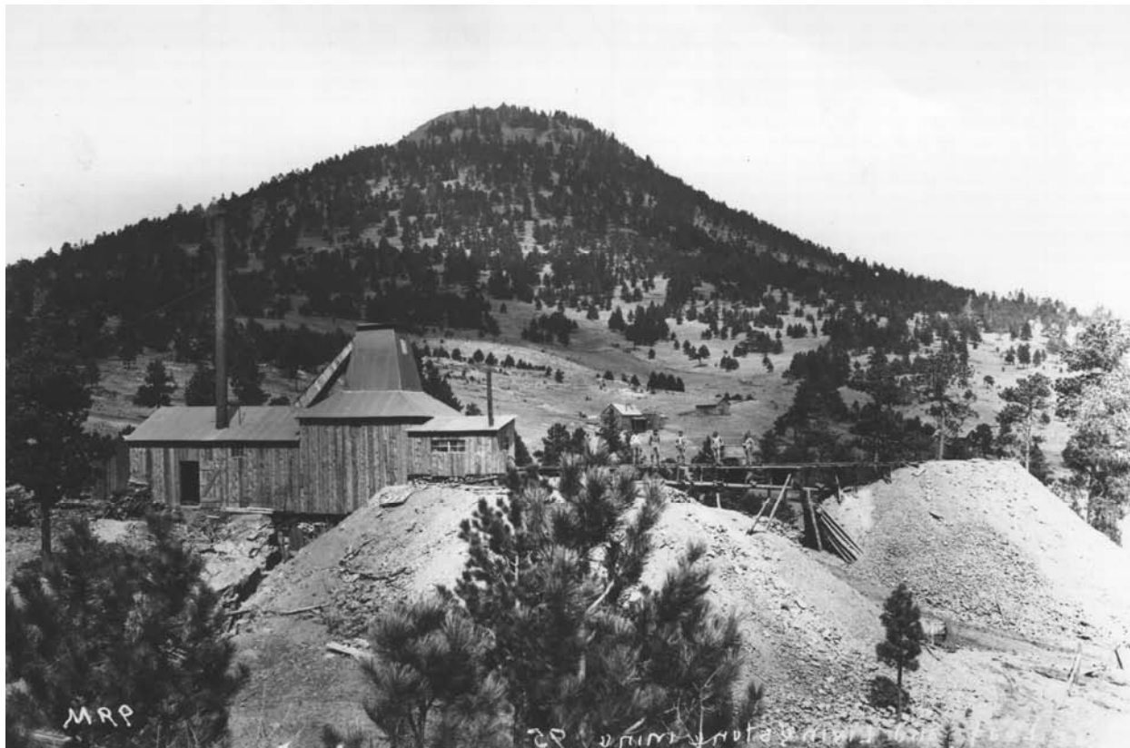
Figure E 4.8.3. The Livingston Mine was one of the Sugar Loaf Mining District's principal producers during the late 1880s and early 1890s. The view is northward toward Sugar Loaf Mountain, in the background. The mine typifies Boulder County's modestly successful shaft operations, and the left portion of the shaft house enclosed a hoist and boiler while the peak stood over a headframe. Source: Boulder Carnegie Library, 219-5-13.
