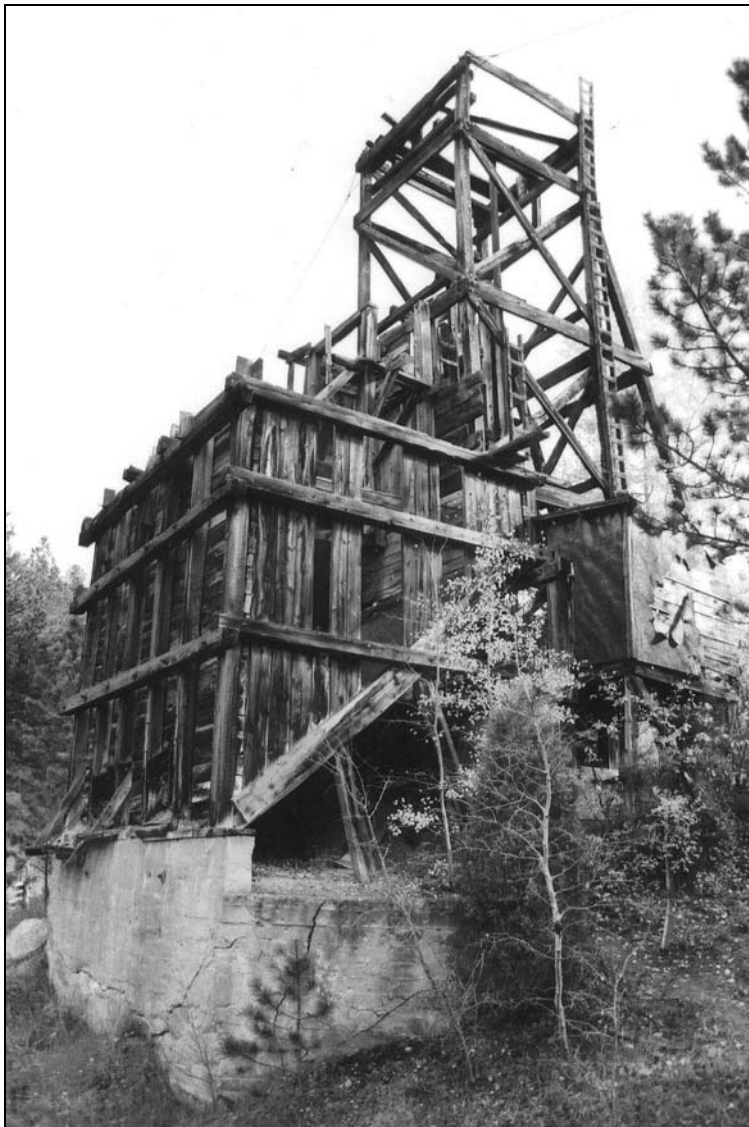
Figure E 5.2.40. The Blue Jay Mine featured a sloped floor ore bin adjacent to the headframe. Most ore bins stood on the shoulder of a mine's waste rock dump. Source: Author.
