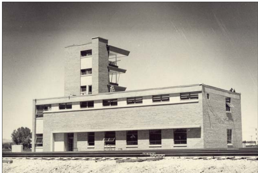
Figure 1. The nearly completed D&RGW rail yard tower shows the influence of the International style in the early work of Wheeler and Lewis. Source: Colorado Historical Society
