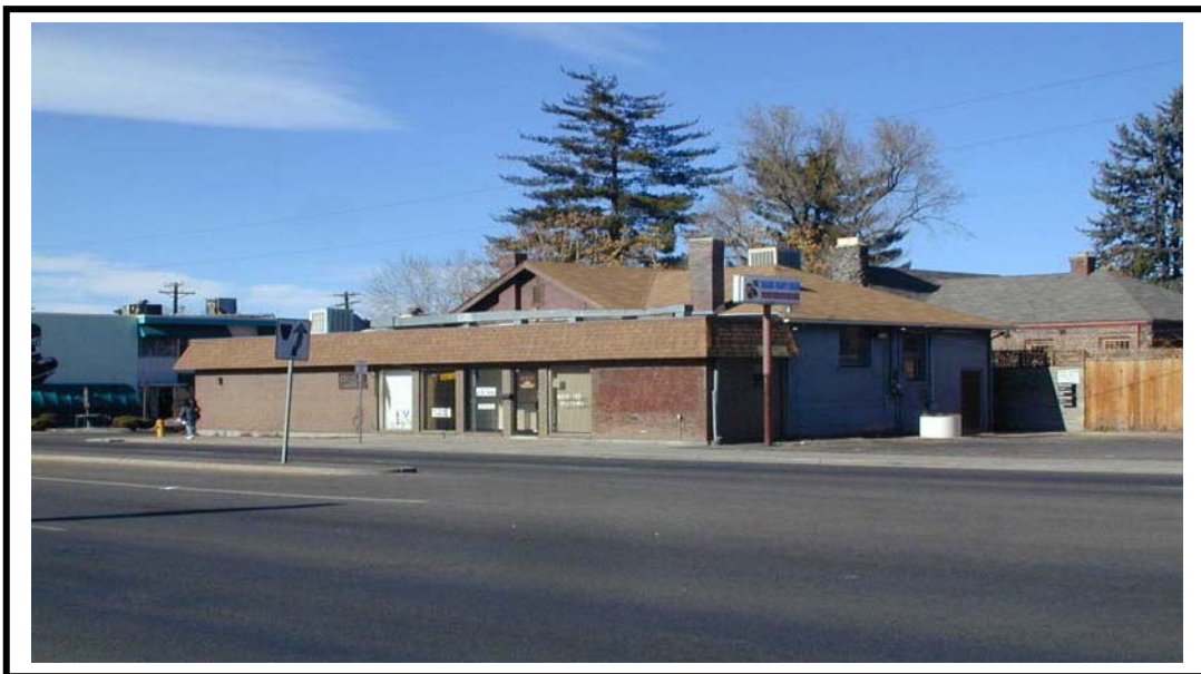
A commercial property on Colfax Avenue in Aurora with a Neo-Mansard addition in front of an existing building.
