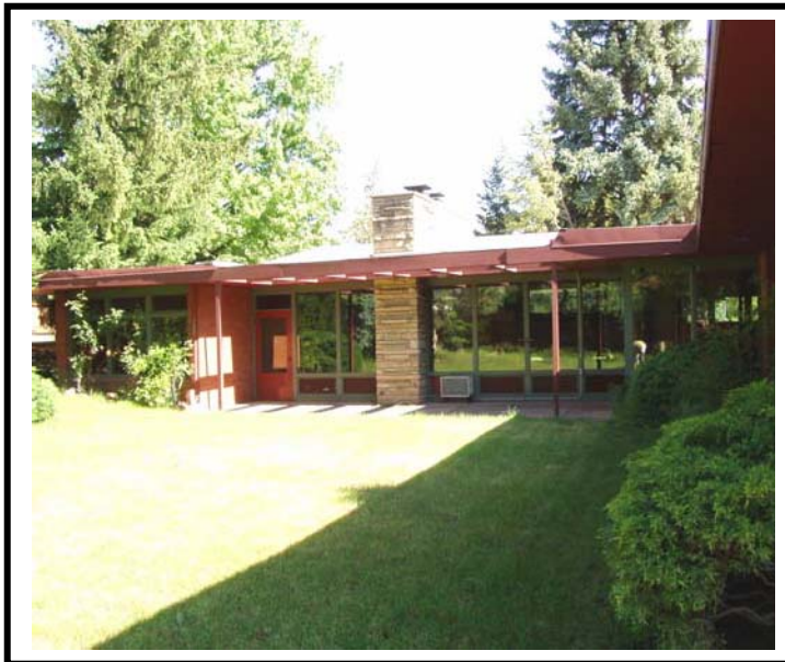
Designed by locally prominent architect James Hunter in 1951, this house in Boulder exhibits many of the features typical of Usonian architecture. Here the rear open side faces south and the chimney integrates the interior and exterior.
