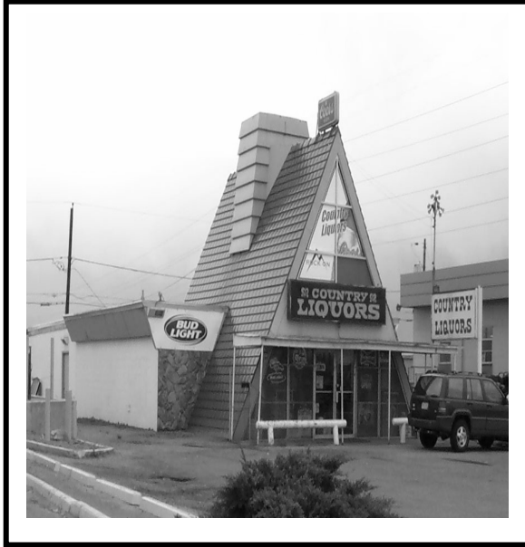
A-frame liquor store with addition, Aurora (Photo courtesy of Lyle Hansen)
