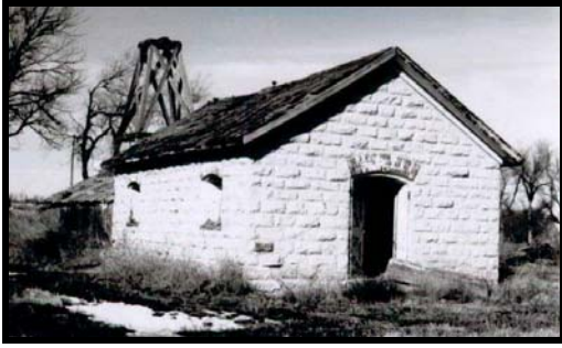
Union Pacific Pumphouse, 1995
