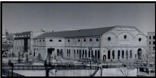
Denver Tramway Powerhouse, 2001
