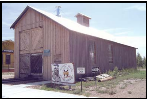
Westcliffe Engine House, 2003
