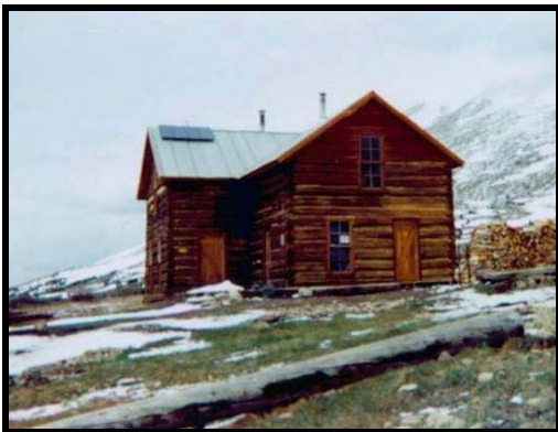
The newly restored Boreas section house in 1998
