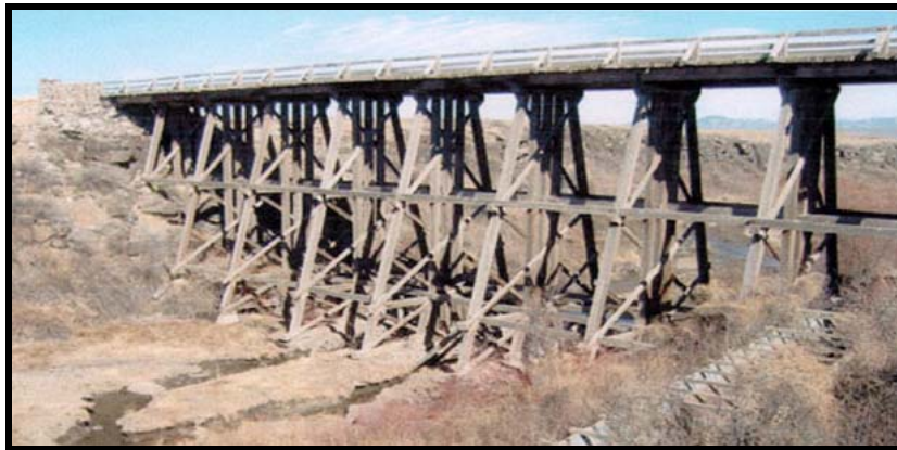
San Luis Valley Southern Railway Trestle, 2002
