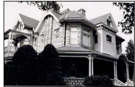
The Baxter House is a good example of the use of native sandstone. (1978)
