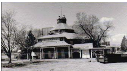
The Elitch Theater recently underwent conversion to a performing arts center. (1988)
