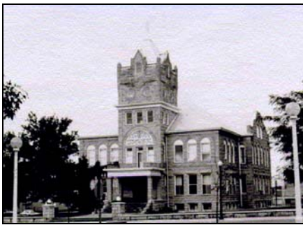
Huerfano County Courthouse continues to serve as the county courthouse. (1973)
