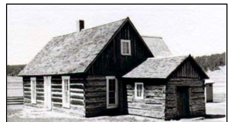
The Hornbek House is a sturdy, well-constructed log building. (1981)
