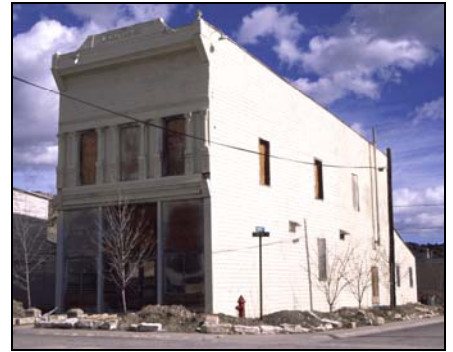
The I.O.O.F. Hall/ Crest Theater exhibits a stone-patterned stamped metal exterior. (1999)
