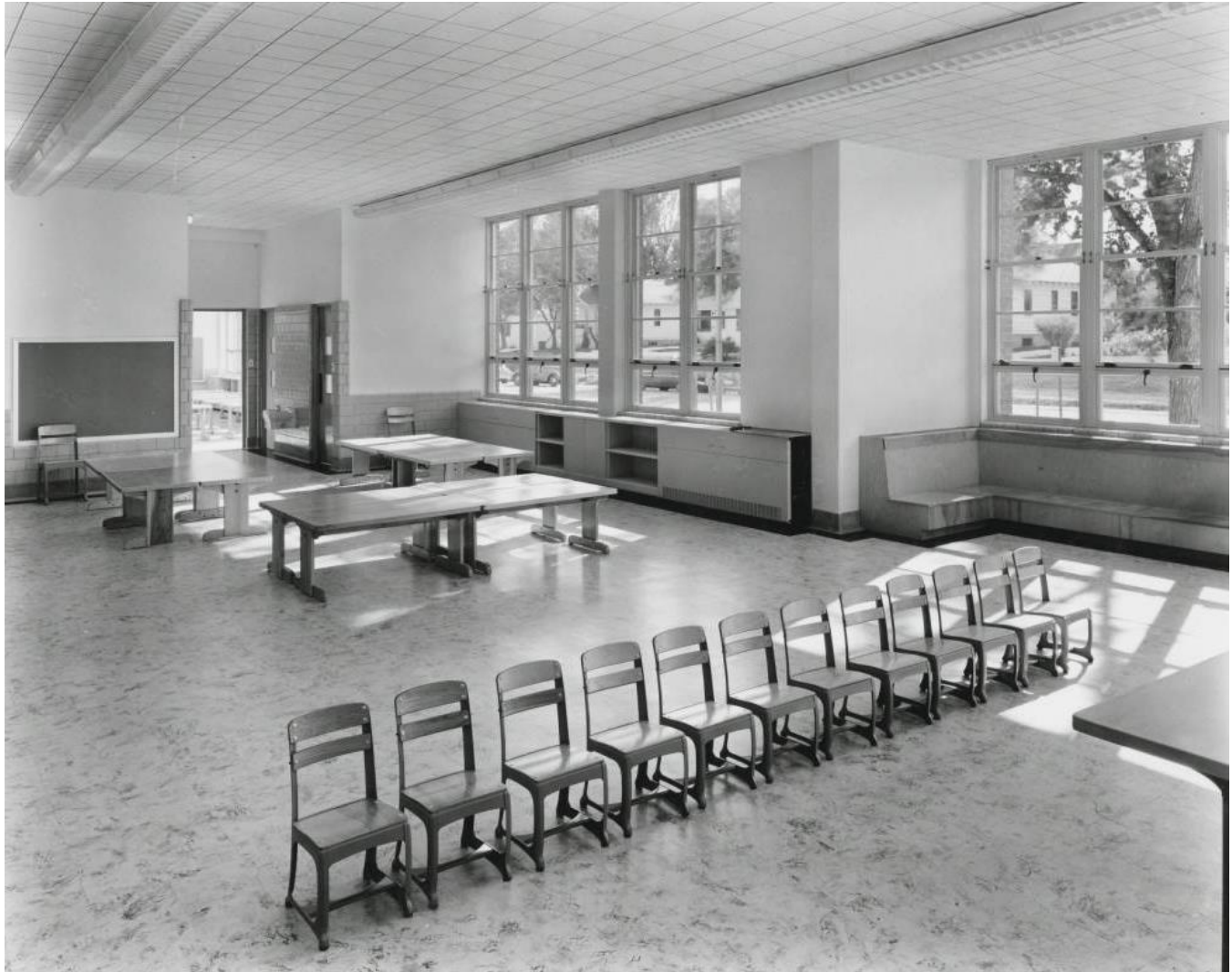
Figure 3. Classroom in Beach Court Elementary School addition, completed 1950. Bright classroom with large bands of windows. Room features acoustic tile ceiling, linoleum floor, movable furniture, built-in seating, and storage underneath windows. (Western History Collection, Denver Public Library. WH1990).
