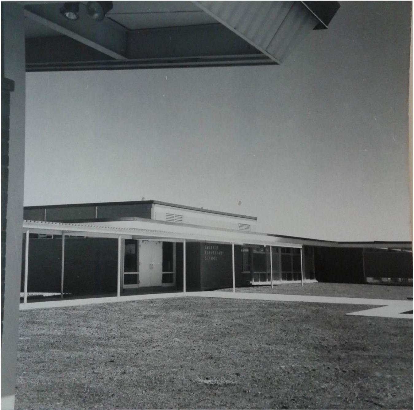
Figure 7. Emerald Elementary School, Broomfield by Wheeler & Lewis, completed 1958. School features sprawling, single-story design, deep eave overhangs, and covered walkways. (Wheeler & Lewis collection, Stephen Hart Library, History Colorado).
