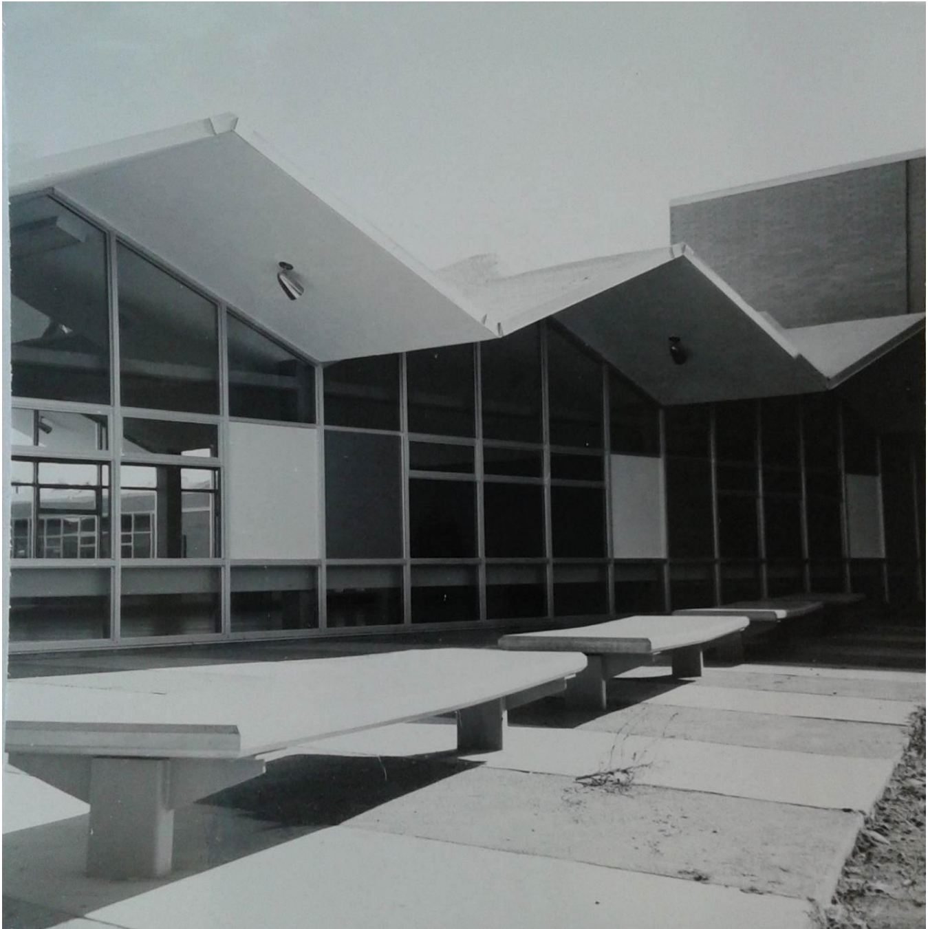
Figure 12. Alameda High School, Lakewood by Wheeler & Lewis, completed 1958. School features folded plate roof. (Wheeler & Lewis collection, Stephen Hart Library, History Colorado).
