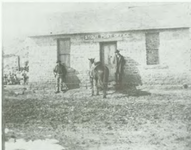
The Stout post office at the Geary ranch.
