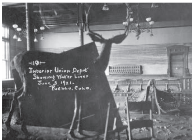
Markings on a wall inside the depot show how high the floodwaters rose. 10036444
