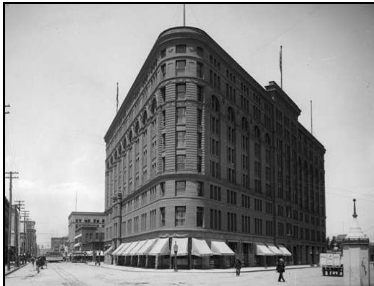
The Boston Building (1889), top left, the Equitable Building (1892), top right, and the Brown palace Hotel (1892), bottom, were important early buildings along 17 th Street which served to draw the Central Business District southeastward. SOURCES: top two, historic postcard views; bottom, Joseph Collier photograph, image C-179, Denver Public Library.
