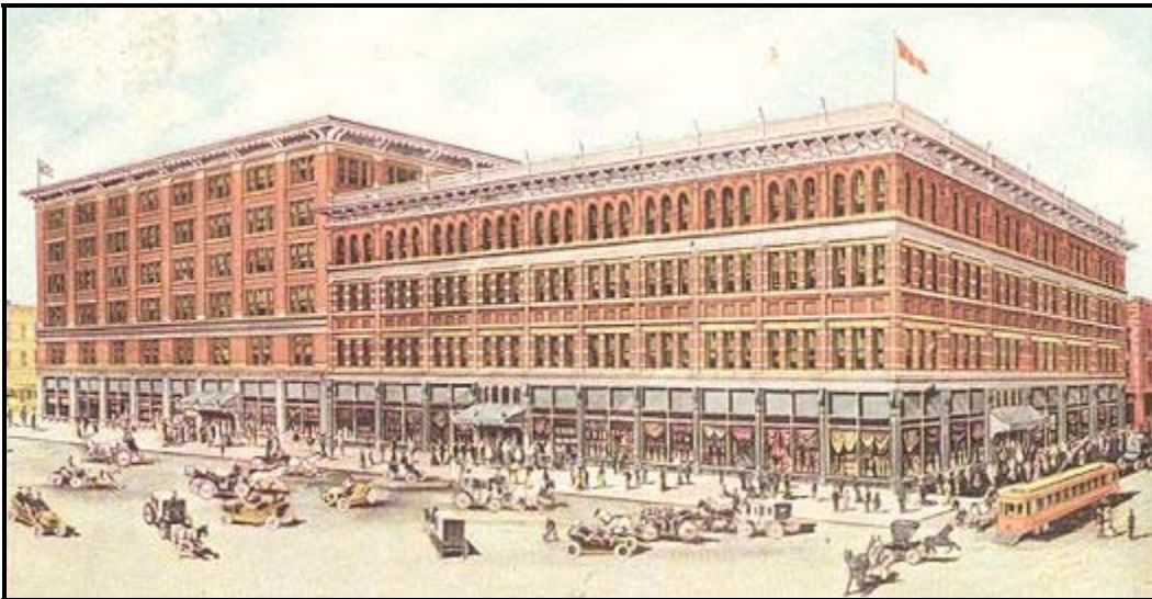
The Denver Dry Goods store (1889, with later additions) at 16 th and California streets was one of several flagship department stores along 16 th Street. SOURCE: historic postcard view.
