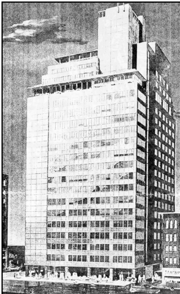
The twenty-three story Denver Club Building at 17th and Glenarm streets was Downtown Denver's first modern high rise building of the postwar period. SOURCE: Denver Club pamphlet, Denver Public Library.
