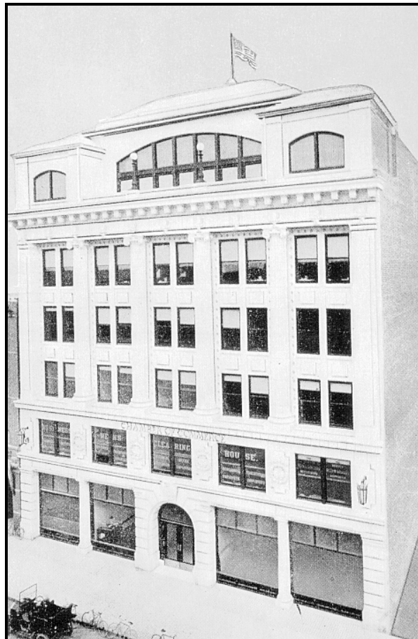
The Chamber of Commerce Building, 1726 Champa Street, was one of several Downtown Denver buildings featuring exterior illumination. SOURCE: historic postcard view.
