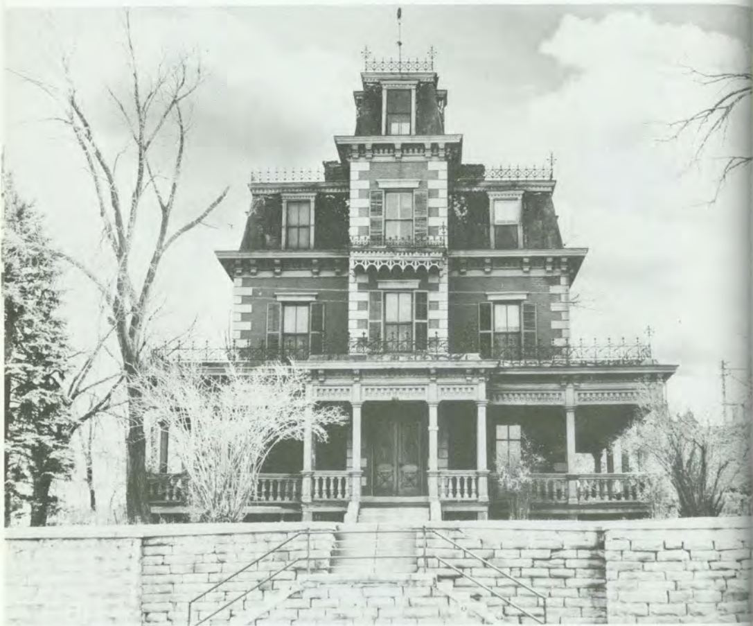
Topped with a cupola, the towering Victorian Rococo Bloom House was built in 1882 by Frank G. Bloom, a Trinidad pioneer who was a merchant, banker, and head of the Bloom Cattle Company. Built of red brick and trimmed with native sandstone, the Bloom House has been restored and furnished in the fashion of the Victorian 1880s. The Baca House next door, built by merchant John S. Hough in 1869 and sold in 1870 to Don Felipe Baca, a successful sheep rancher, has been restored to reflect the life style of a prosperous Hispano family during the 1870s.
