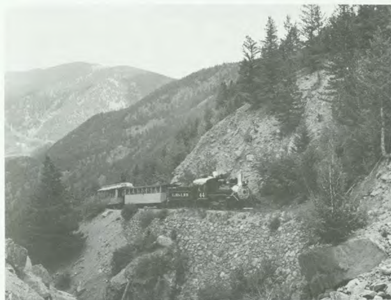
The Georgetown, Breckenridge, and Leadville Railroad chugs along the reconstructed track of the Georgetown Loop, once advertised as the "Scenic Wonder of the World."
