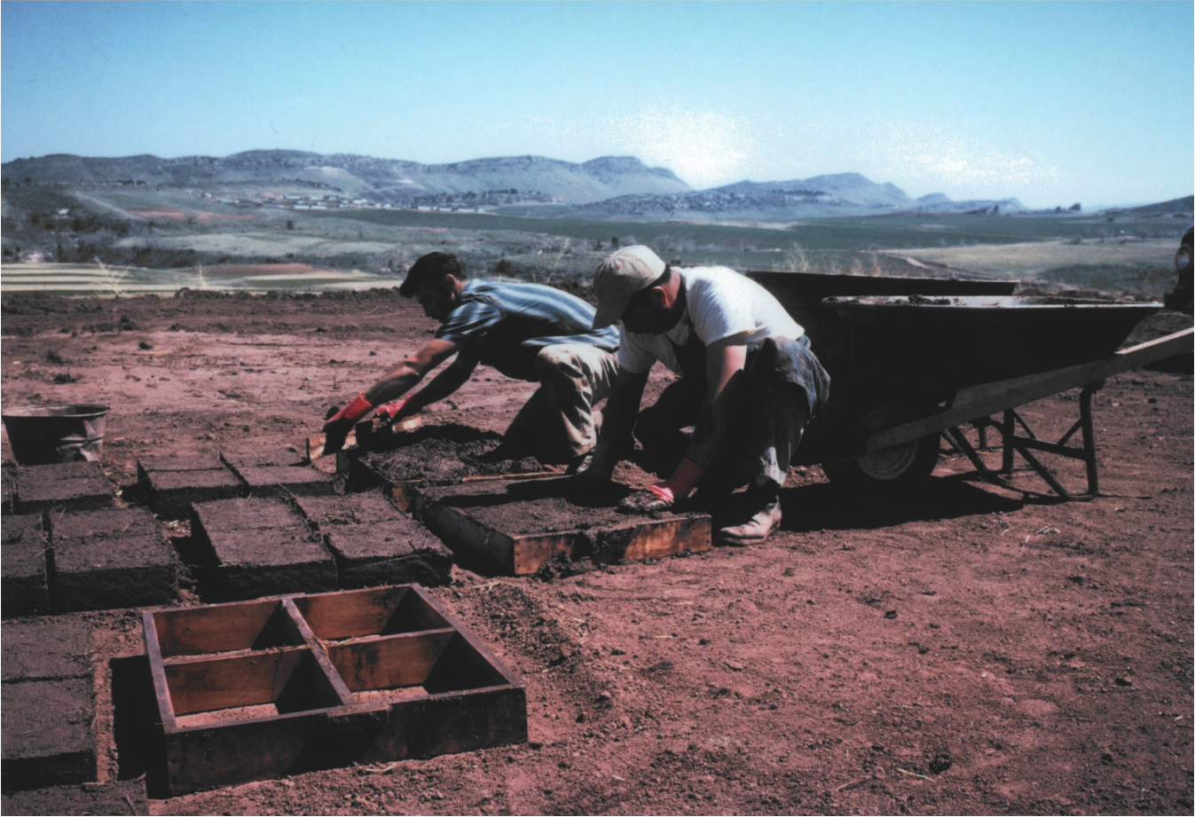
H2. Adobe brick-making. View southeast, ca. 1962-63. Collection of Holly Arnold Kinney.
