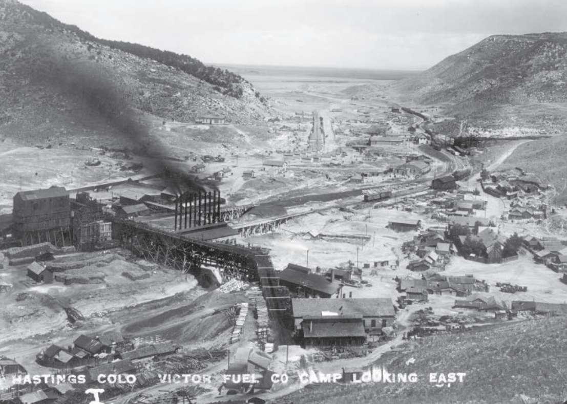
An aerial view shows the coal camp of Hastings and its tipples, washer, and screening plant. Company houses line the road that cuts east through the canyon toward Ludlow. 20004914
