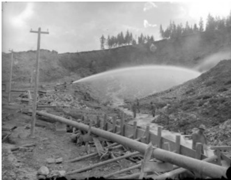
Fig.E.II.3 Hydraulic placer mining at Gold Run Mine, Breckenridge, Summit County, between 1880 and 1890. A high-pressure jet of water, emitted by a monitor against gravel banks, washes the gravel through a system of sluices. Hydraulic mining required capital, advanced hydraulic engineering, and extensive claim holdings. Denver Public Library, Western History Collection, X-60113.
