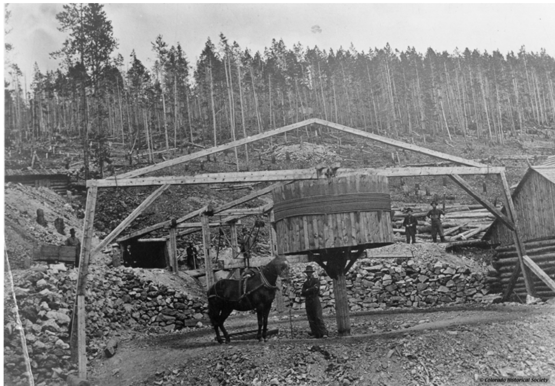
Fig. E.I.4 A single-horse powered whim provided hoisting power for an 1860's hardrock mine. Location unknown. Collection of the Stephen Hart Library, Colorado Historical Society.
