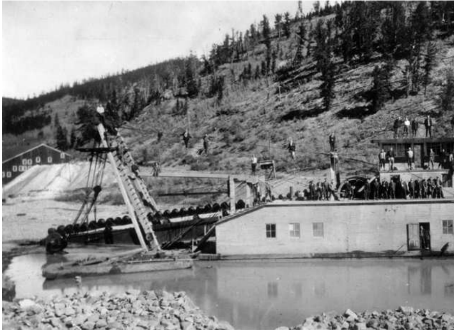
Fig. E.II.6 The Reliance dredge's bow, possibly in 1906. This features the bucket-line for excavating gravel. The gantry and cables controlled the heavy bucket-line's elevation. The bucket-line delivered gravel to processing machinery in the superstructure. Denver Public Library, Western History Collection, X: 60161.
