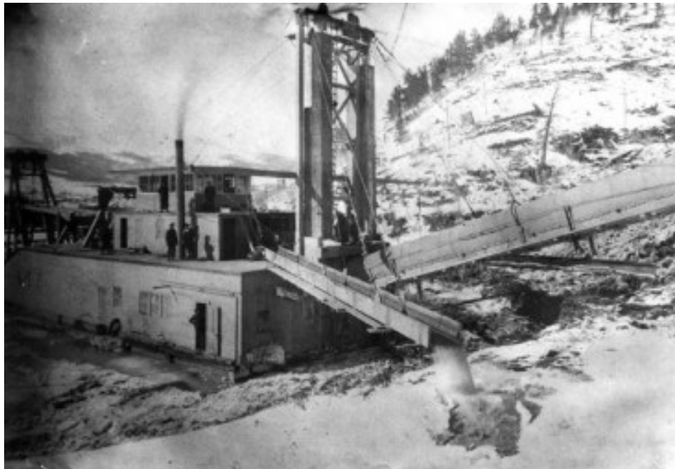
Fig. E.II.5 The stern of the Reliance dredge, at the mouth of French Gulch during winter in 1905. The tailings stacker, braced by the tall gantry, extends right and features a canvas shroud to prevent freezing. Water from processing pours out of the flume at center. Denver Public Library, Western History Collection, X: 60156.
