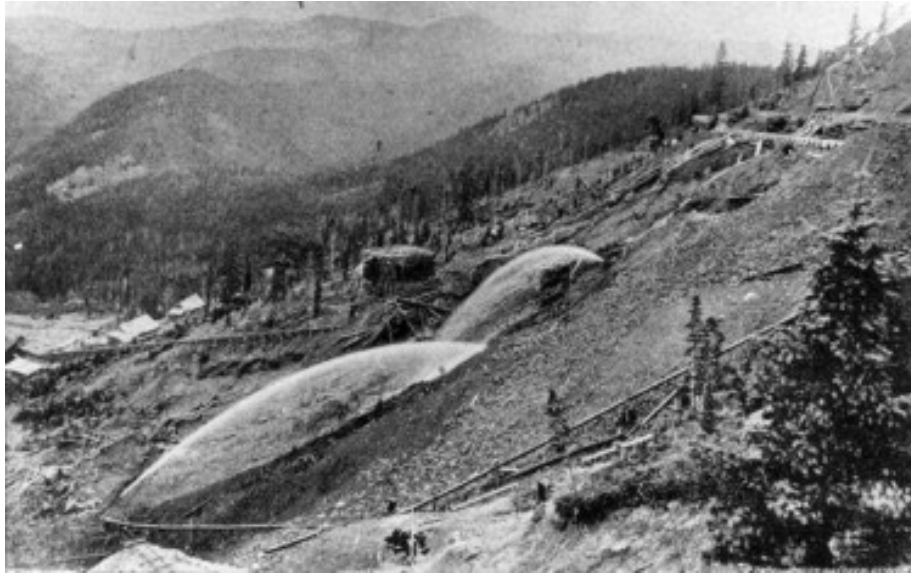
Fig.E.II.2 Hydraulic placer mining at French Gulch, Summit County, 1897. Heavily capitalized companies dominated placer mining by the late 1870s and employed advanced engineering to work bench deposits that offered disseminated gold. Denver Public Library, Western History Collection, Williamson-Haffner, X-60193.
