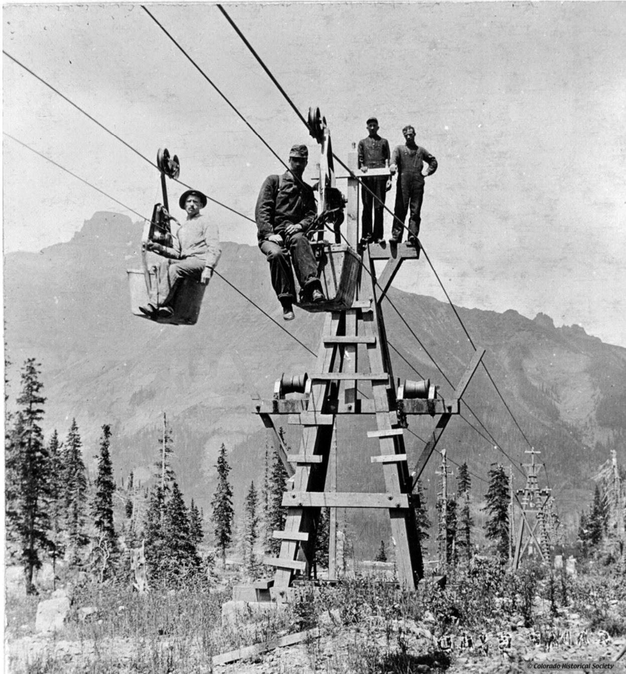
Fig. E.I.16 Camp Bird Aerial Tramway, near Ouray, Colorado, about 1910. Collection of the Stephen Hart Library, Colorado Historical Society.
