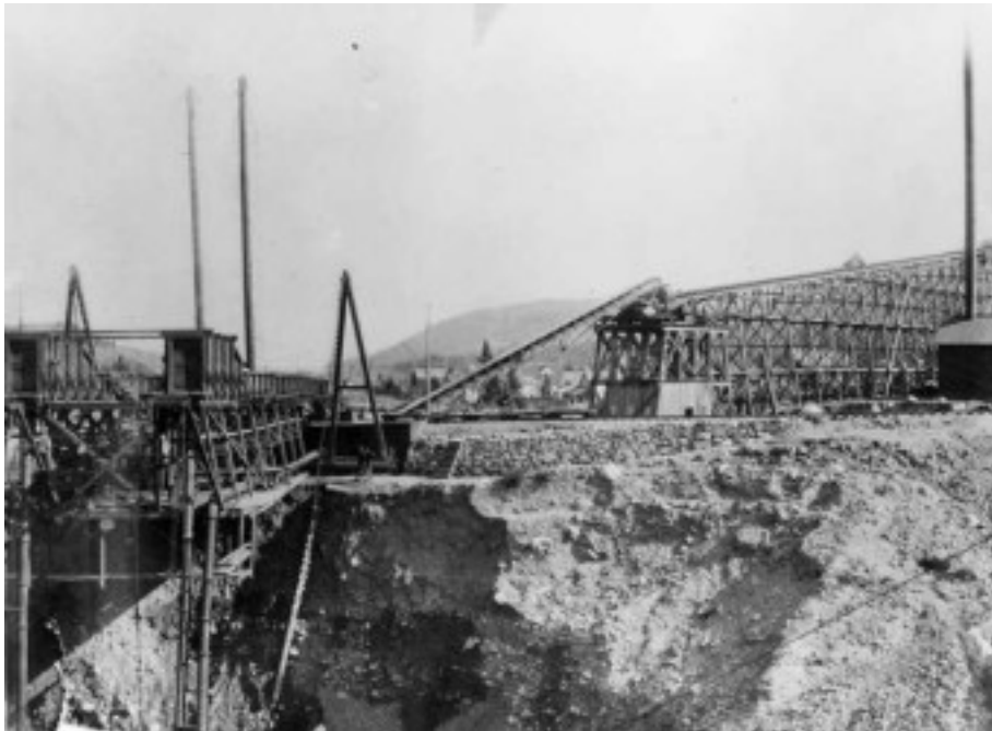
Fig. E.II.4 Deep-pit mining at Gold Pan Pit, near Breckenridge, Summit County, between 1900 and 1913. Engineers and investors long suspected that rich placer gold lay along the bedrock floors of the Blue River near Breckenridge. By around 1900, several companies employed advanced engineering to remove the gravel in deep pits, as shown here. Conveyors carried overburden gravel to tailings dumps and hydraulic suction elevators, supported by timber structures, siphoned gold-bearing material and dumped it into sluices. Operating costs exceeded profits at most pits. Denver Public Library, Western History Collection, X-62420.
