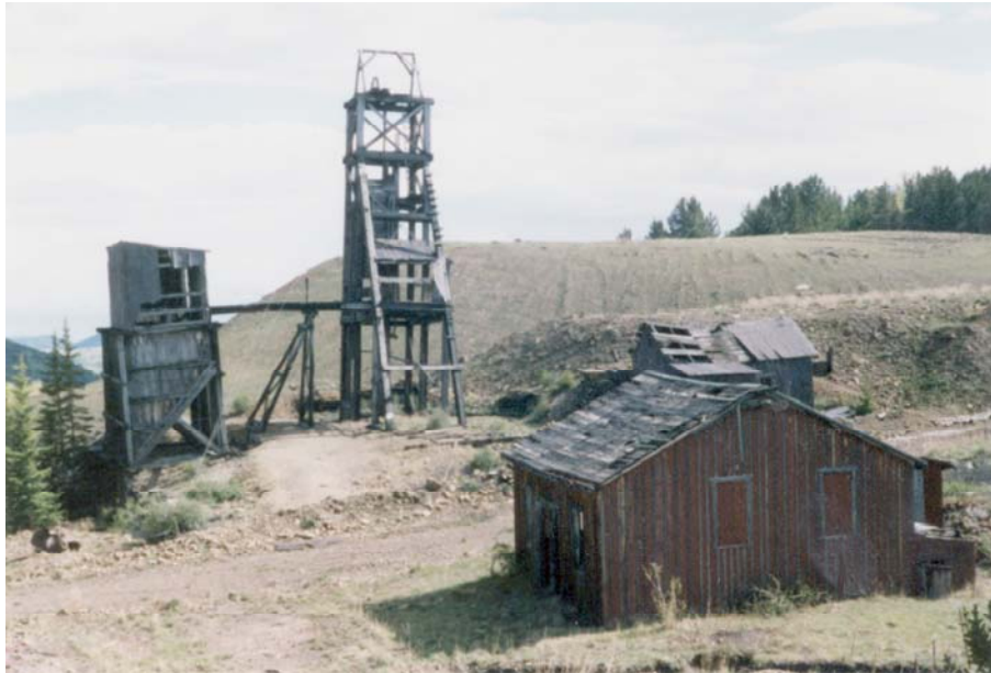
Fig. E.II.15 Surface plant components at the Joe Dandy Mine, Cripple Creek. The surface plant components of large mines were often housed in individual buildings. This practice had extended to most smaller shaft mines by the 1910s when the U.S. Bureau of Mines outlawed shaft houses. The headframe (a four-post derrick), stands in the open and denotes the shaft. A hoist house enclosed the hoist and a workshop. It stands at lower right. A blacksmith and machine shop is visible slightly above the hoist house, and an ore-sorting house is left of the headframe. Note the trestle linking the ore-sorting house and second landing in the headframe. Eric Twitty, taken 1998.
