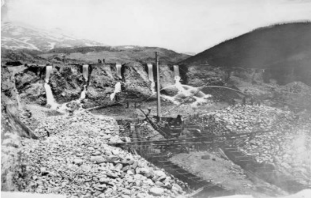
Fig E.II.1 A stream placer near Hoosier Pass, Summit County, around 1880. Organized placer companies employed engineering and capital to work stream placers. Ditches provided water for booming, which relied on a torrent to carry gravel through systems of sluices. Some operations also used derricks to hoist large boulders, exemplified by the structure between the sluices. When workers cleaned gold from the sluices, they shoveled the excess sediment out. In this photo, workers piled it between the sluices. Denver Public Library, Western History Collection, X-60097.
