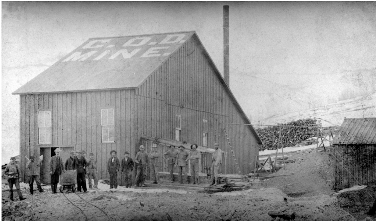
Fig. E.II.13 The C.O.D. Mine, Cripple Creek, during the mid-1890s. This is an example of a typical shaft house for a small, productive mine. The headframe stood underneath the building's high point and the smokestack denotes the location of the hoist. Note the mine rail line exiting the broad doorway. The shaft house also probably enclosed a blacksmith shop and an area where miners dressed timbers. A stack of cordwood in the background served as boiler fuel, and an office and storehouse stands at right. Colorado Historical Society, F-44120.
