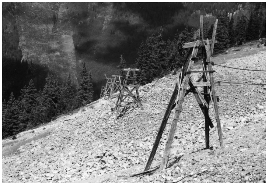
Fig. E.II.52 Aerial tramways featured towers that supported cables for tram buckets. The Pennsylvania Mine, Peru Creek, Summit County, featured a double-rope reversible system in which two buckets ascended and descended the cables in a balanced fashion. The towers are pyramid types. Eric Twitty, taken 1998.
