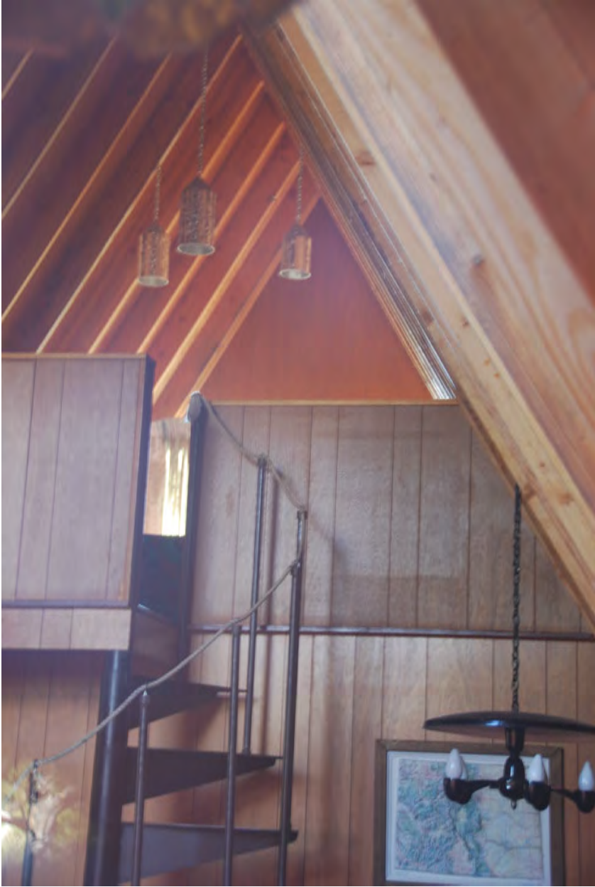
128 Cabin Creek Photo by J. Wahlers 11/2/2017 Interior View
