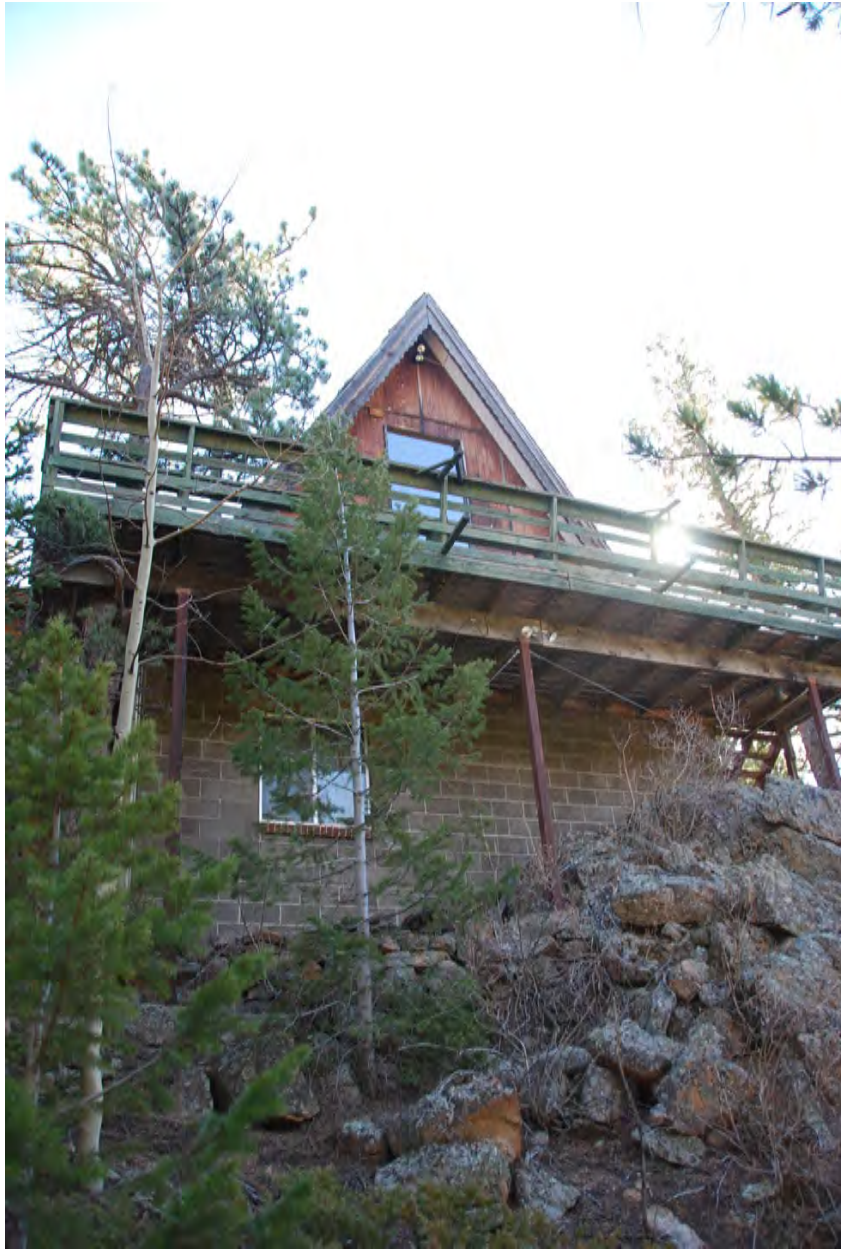
128 Cabin Creek Photo by J. Wahlers 11/2/2017 View of front elevation from below
