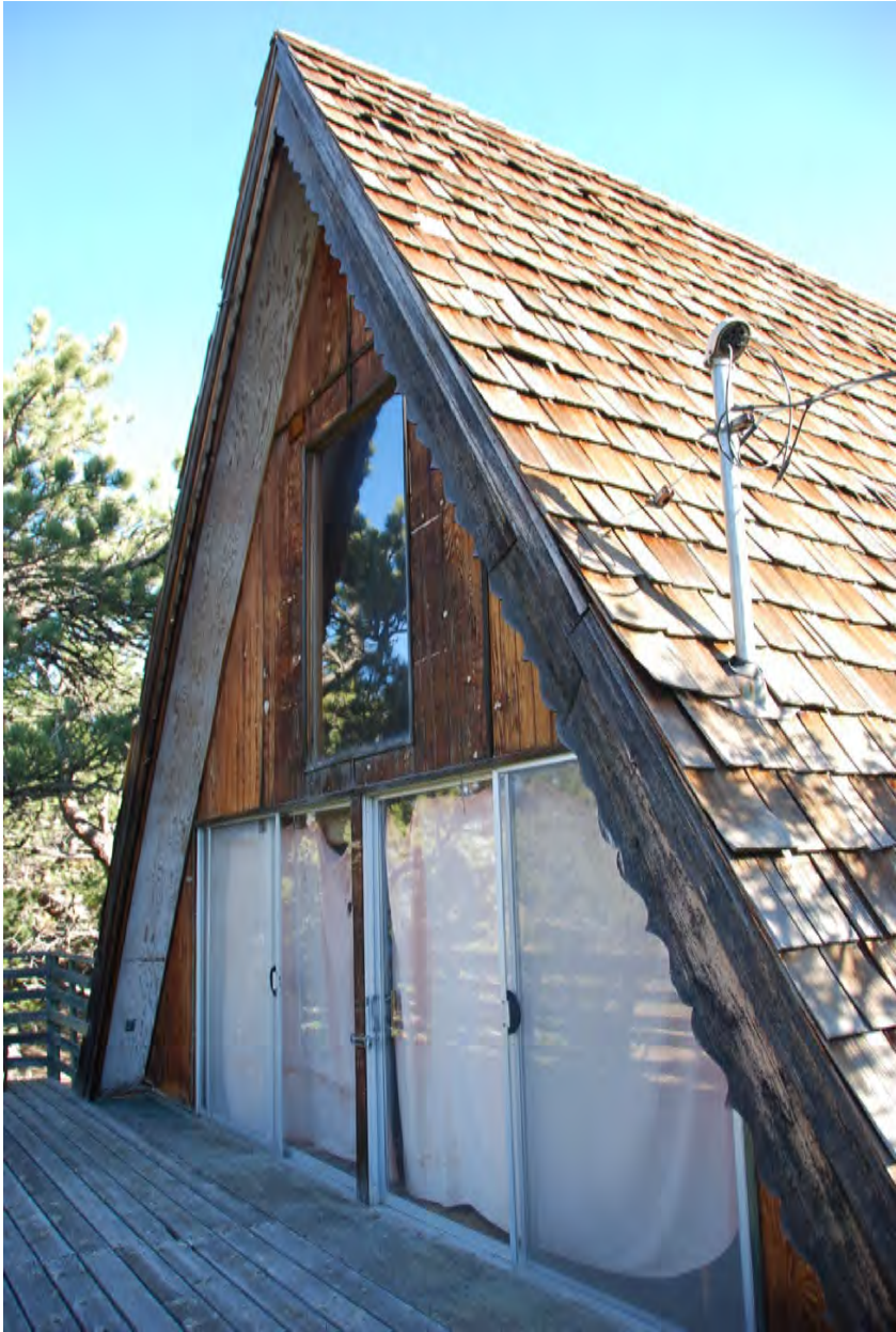
128 Cabin Creek Photo by J. Wahlers 11/2/2017 Front elevation
