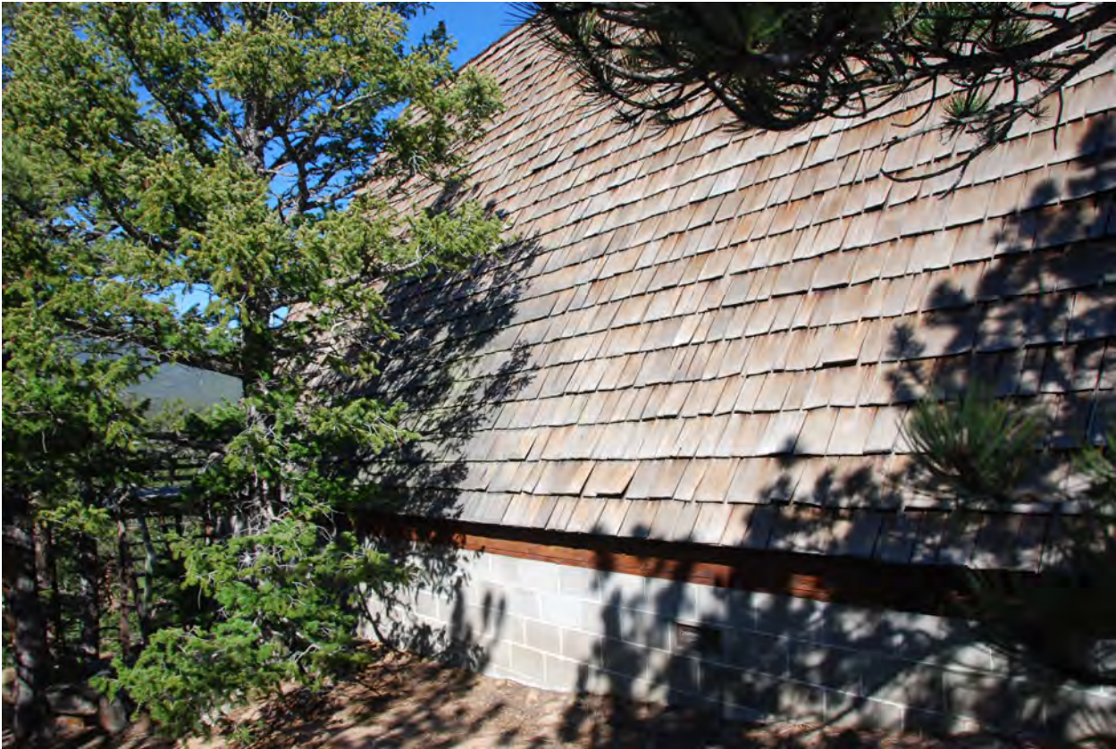
128 Cabin Creek Photo by J. Wahlers 11/2/2017 Side elevation showing concrete block foundation
