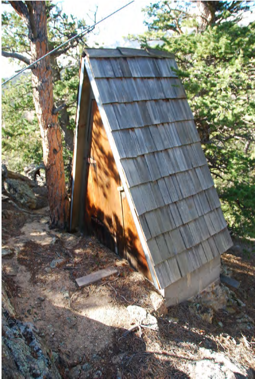
128 Cabin Creek Photo by J. Wahlers 11/2/2017 A frame outhouse
