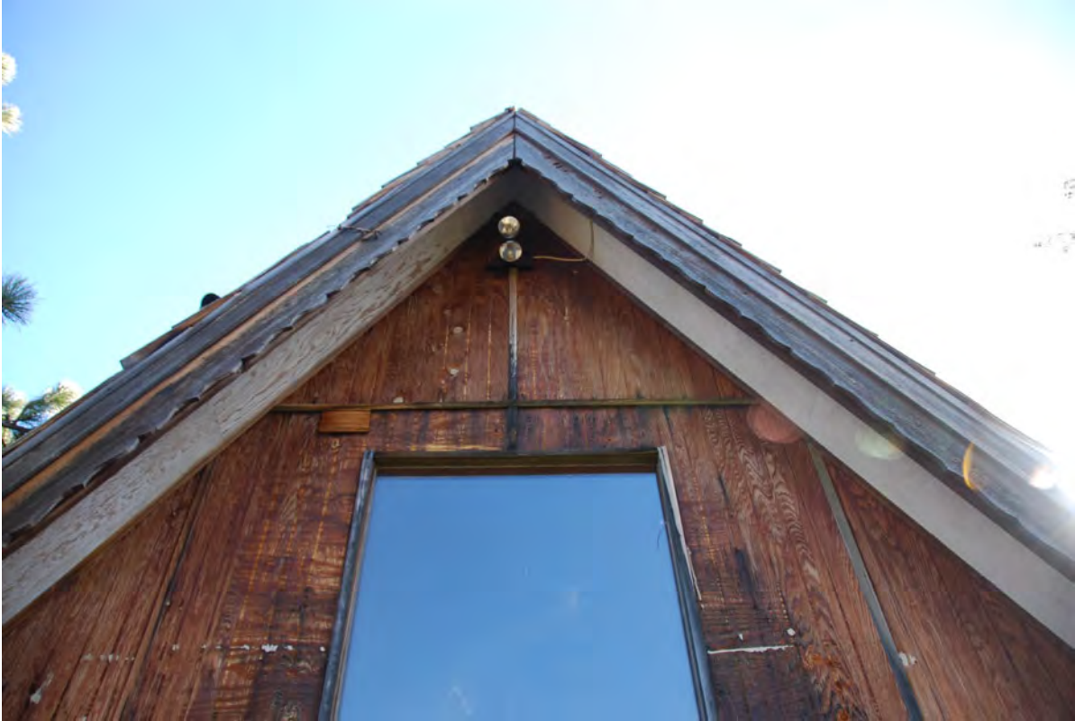
Detail of bargeboard and paneling
