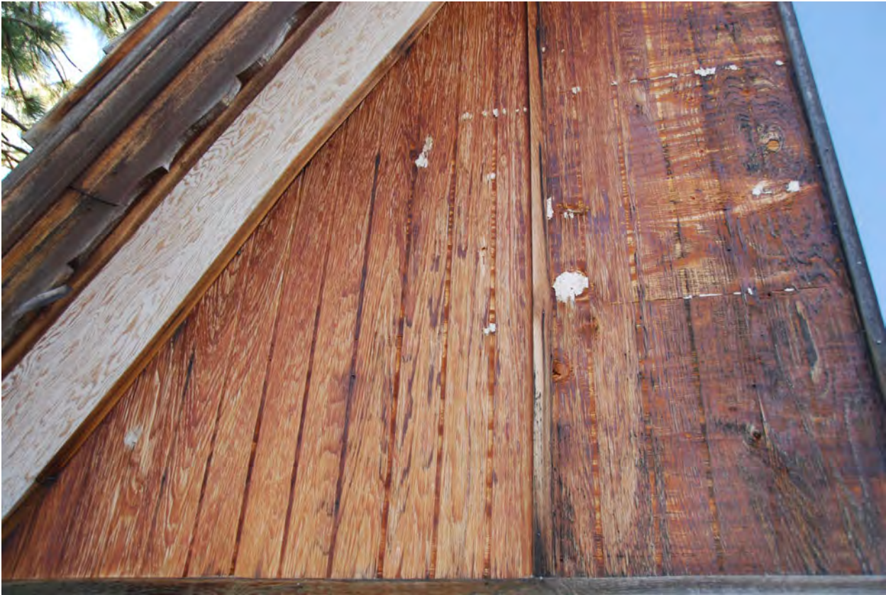
128 Cabin Creek Photo by J. Wahlers 11/2/2017 Paneling that gives impression of board and batten
