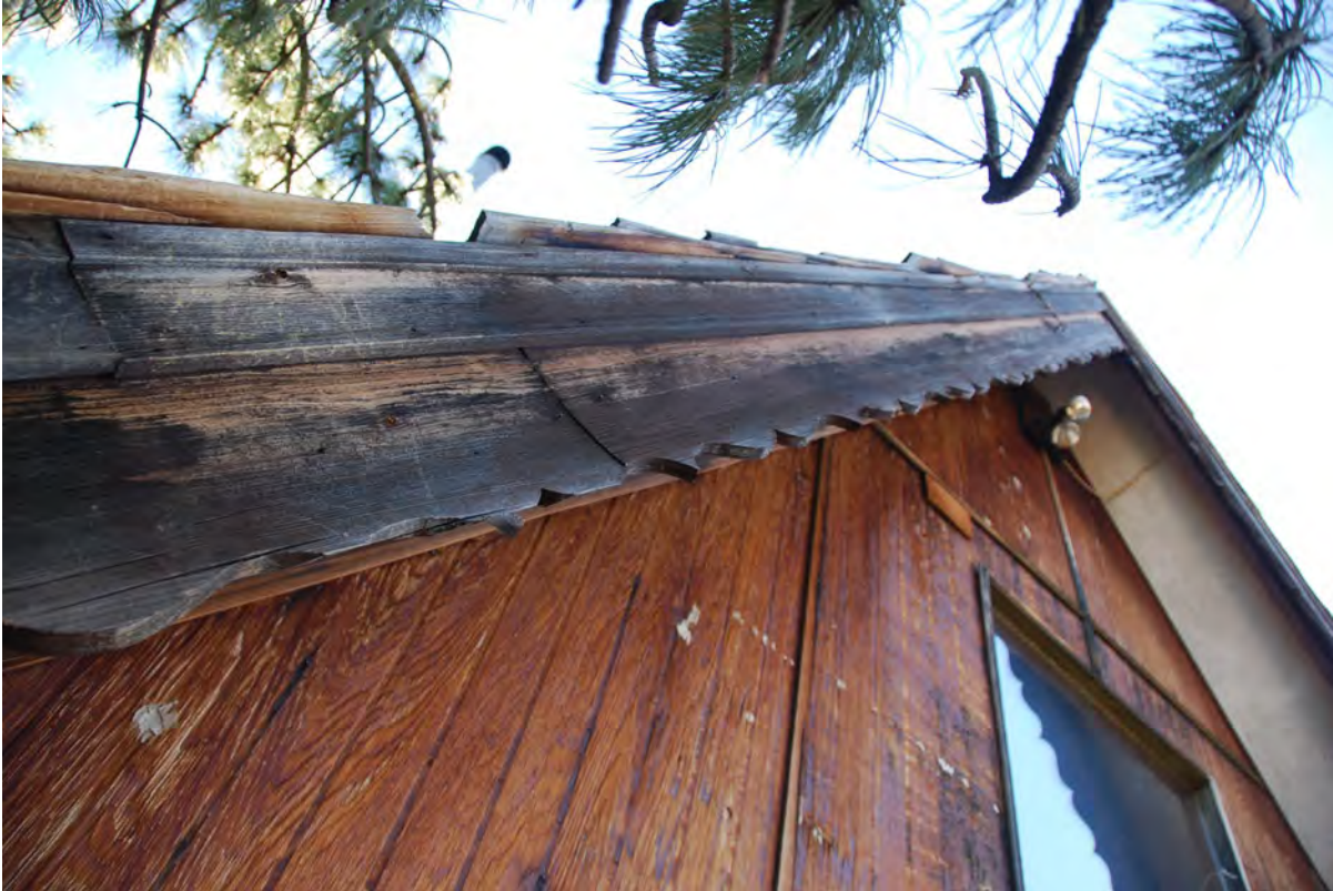
Detail of bargeboard and paneling
