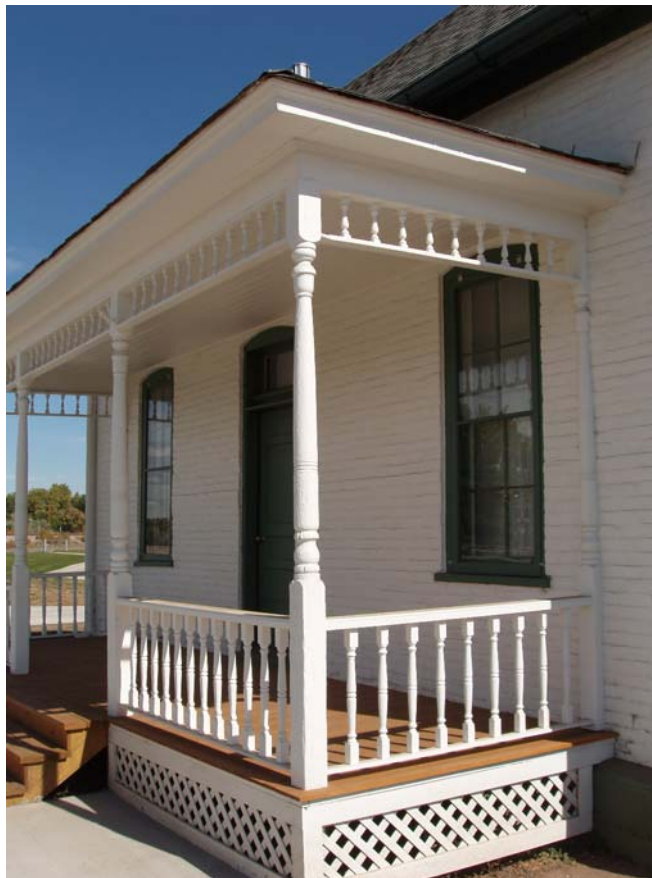
Photo 2 Southeast side of porch, camera facing northwest*
