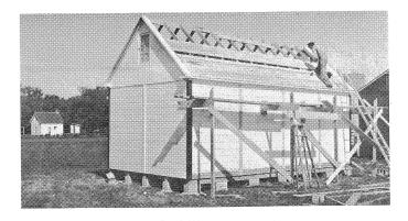
through the roof. Removing the old roofing reduces roof weight, permits securely fastening new roofing to the roof framework and replacement of rotted roof boards or purlins where needed.
