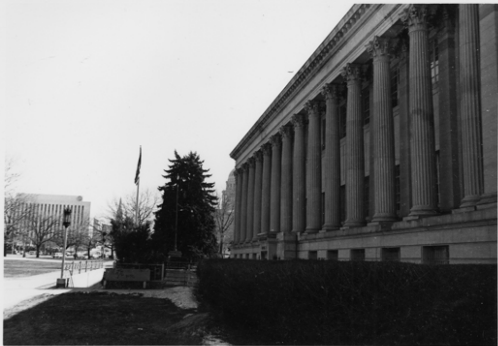
5DV.161.4 Water Board Bldg.
