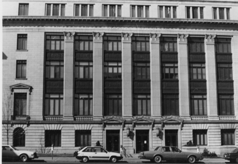
5DV.161.4 Water Board Bldg.
