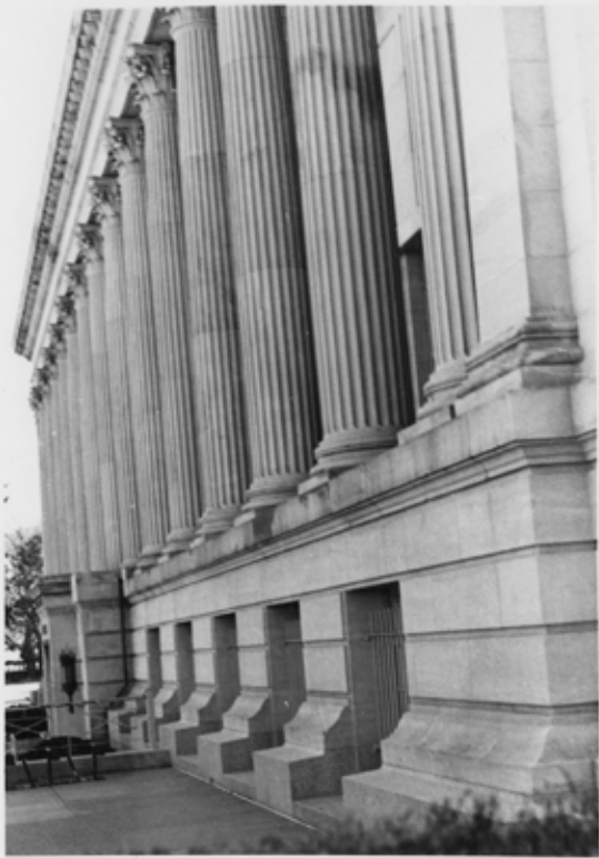
5DV. 161.4 Water Board Bldg.
