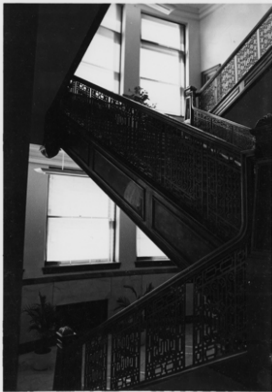
5DV. 5990 State Museum Bldg. Staircase
