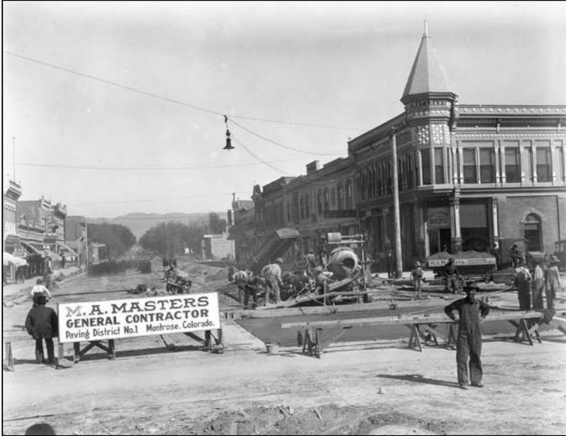
**Figure 28.** The sign reads "M. A. Masters General Contractor Paving District No. 1 Montrose, Colorado." The firm is paving Main Street in Montrose. A crew is leveling concrete being poured from a mixer, while others haul rock and dirt in wheelbarrows. Main Street in 1919 formed a part of the Rainbow Route through western Colorado. Source: Denver Public Library, Western History Department.
