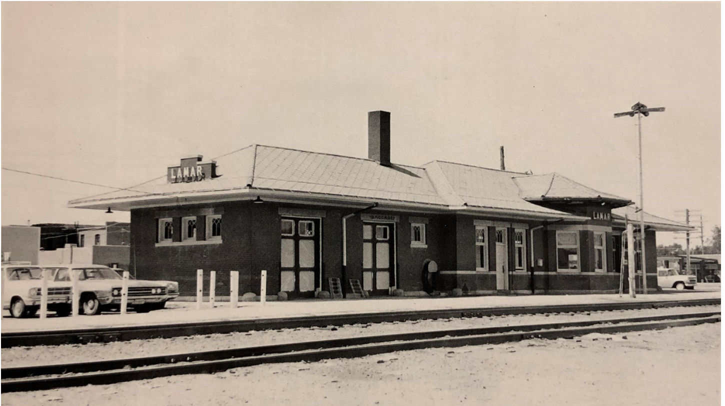
Figure 12: Lamar depot in 1973. (Source: Pounds, Santa Fe Depots, the Western Lines /Collection of Harold K. Vollrath)
