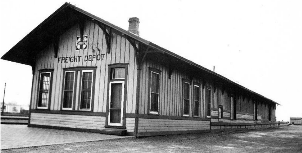
Figure 6: AT&SF Freight Depot in 1931. Based on its size and design it is likely that this building is the 1888 combination freight and passenger depot documented on the 1906 Sanborn Map, moved and repurposed in 1907 to handle freight services only. (Kansas Historical Society)
