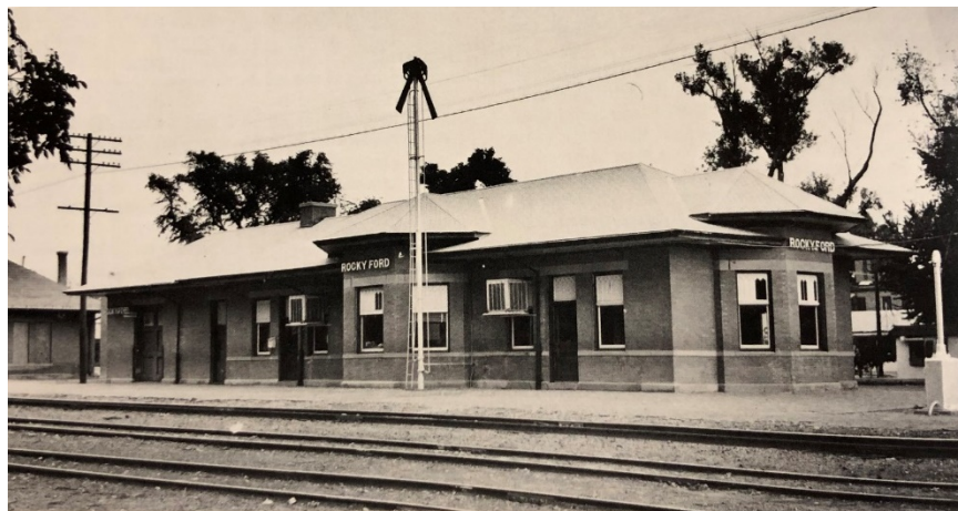
Figure 10: The AT&SF passenger depots in Garden City, Kansas, (top) Las Animas, Colorado, (5BN.415) (middle) and Rocky Ford, Colorado, (5OT.190) (bottom), followed the same standardized design as the Lamar depot with some minor variations. (Source: Pounds, Santa Fe Depots, the Western Lines /Finney County Historical Society/John McCall Collection/Frank O. Kelley Collection)
