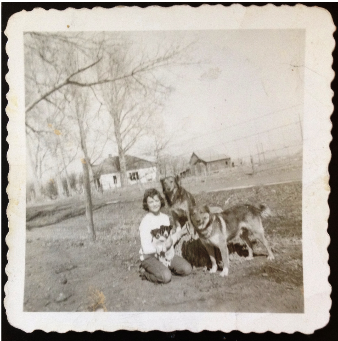
Figure 2: View of 330 N Taft Hill Road property from across the street in 1955. Source Karen Lake.
