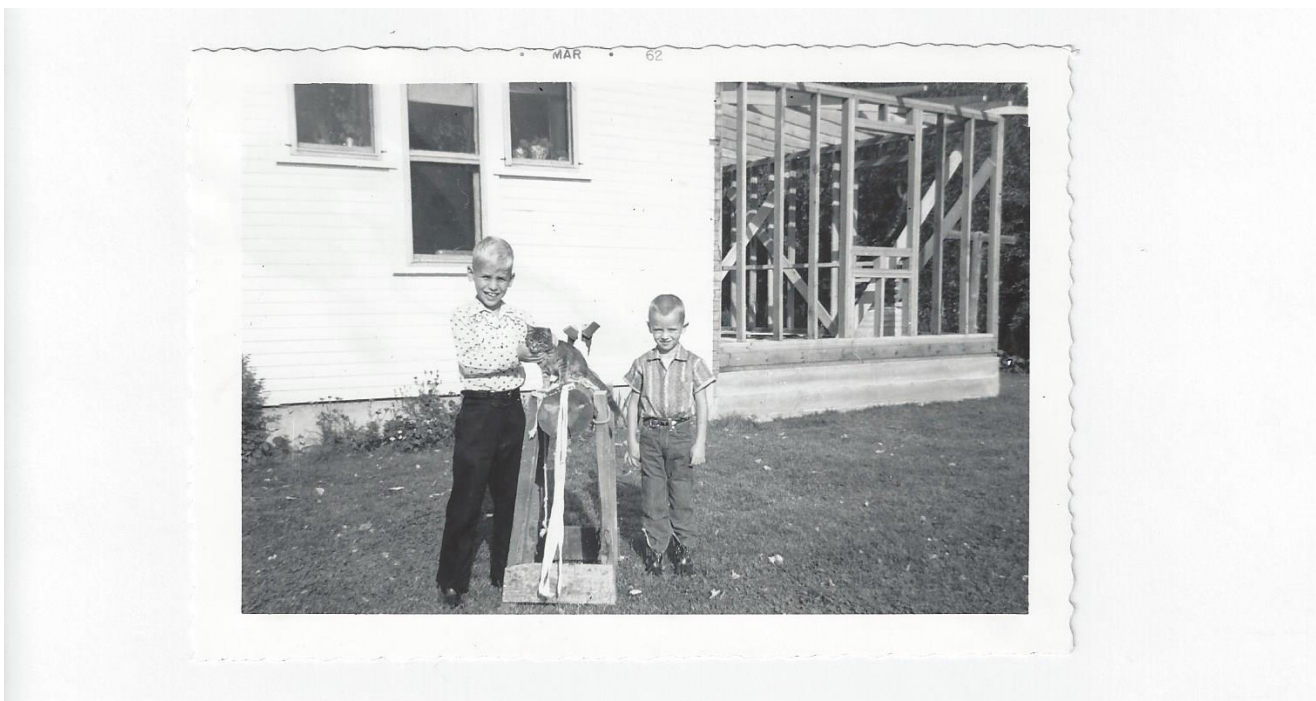
Figure 8: Photo courtesy of John Lee Slagle, dated March, 1962. View is of the east side of the house with framing of the addition visible. John is pictured on the left and his brother on the right.
