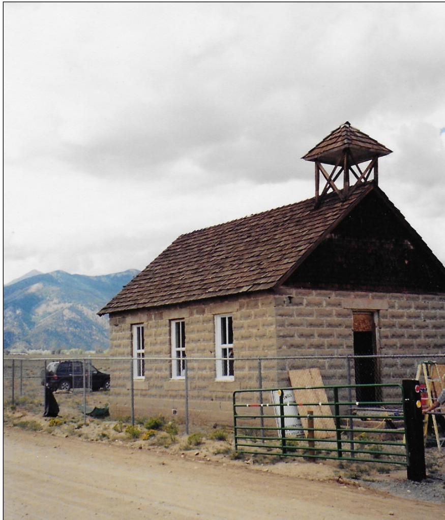
Figure 7. This view northwest taken at the time of the ca. 2001-02 rehabilitation project and shows the two-over-two-light wood replacement windows. SOURCE: Colorado State Land Board.
