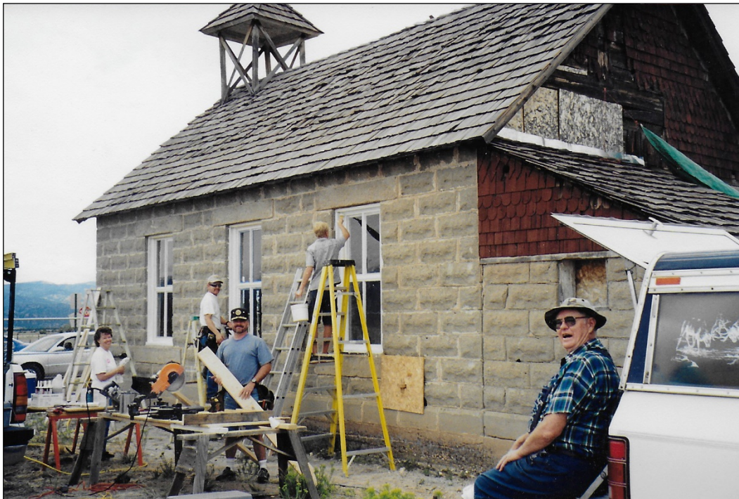
Figure 6. A local effort to rehabilitate the school is underway in this ca. 2001-02 photograph (view southeast). The project included replacing the windows and shingling gable faces. SOURCE: Colorado State Land Board.
