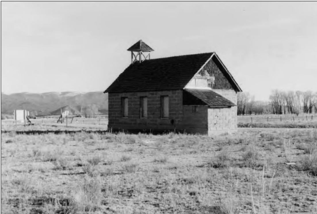
Figure 5. The rear and north wall of the school is shown in this ca. 1998 view. SOURCE: Kelly, Mount Princeton School, survey form, 1998.
