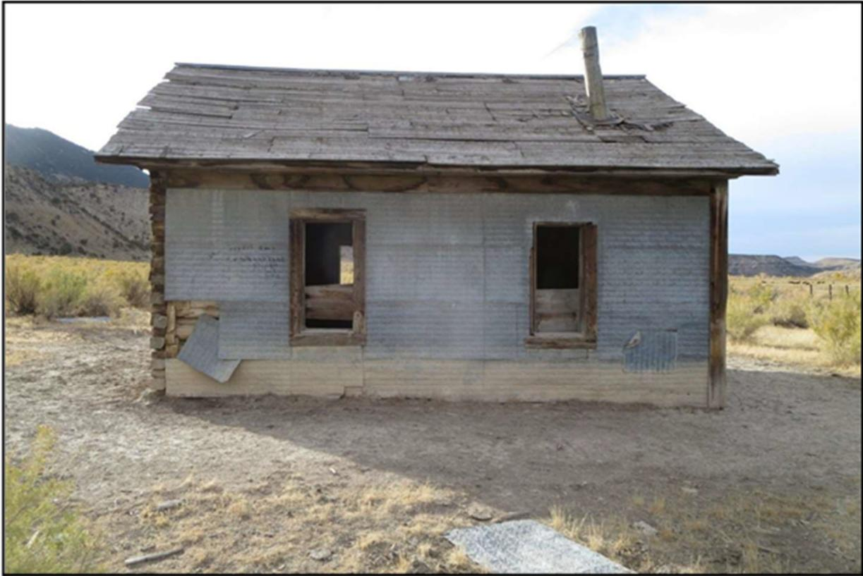
Plate 2. Eastern façade showing roof without shingles in 2020. Looking west, Photo 12.
