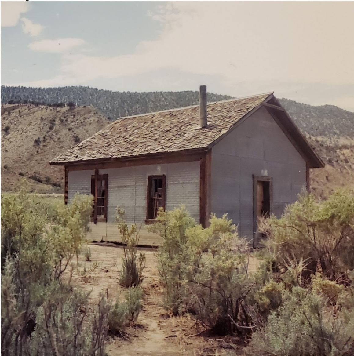
Plate 1. Oblique view of Yellow Creek Schoolhouse showing north and east facades and wood shingles on roof. Looking southwest. 1989 photo by Robert B. Watson on file at White River Field Office, Bureau of Land Management.
