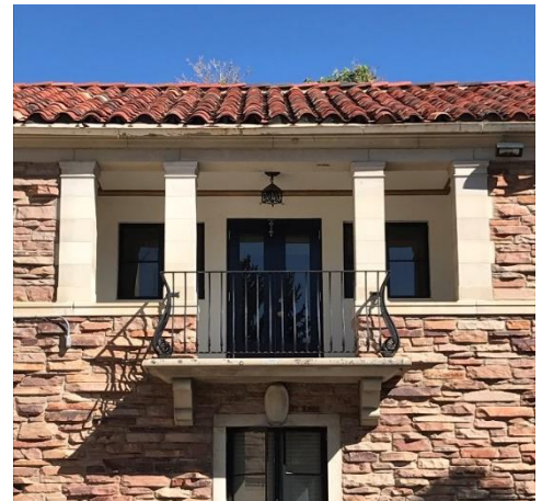
4. Sewell Hall, U of Colorado Boulder photo: M.
