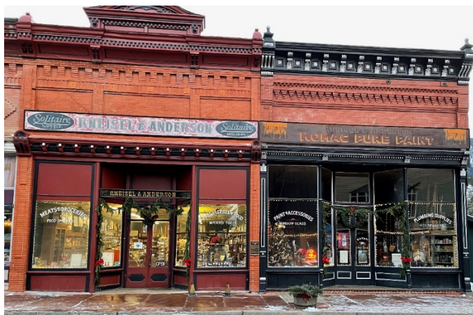
Kneisel & Anderson and Spruance Buildings, Clear Creek County
