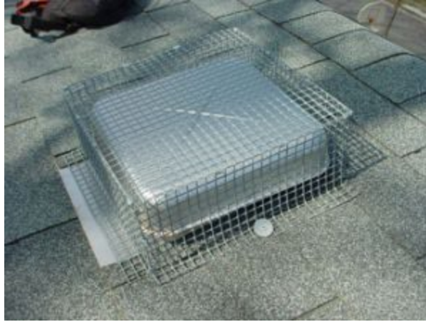
Figure 36: Roof Vent with Retrofitted Wire Mesh Cover (Roof Vent Screens Installation, 2023)
