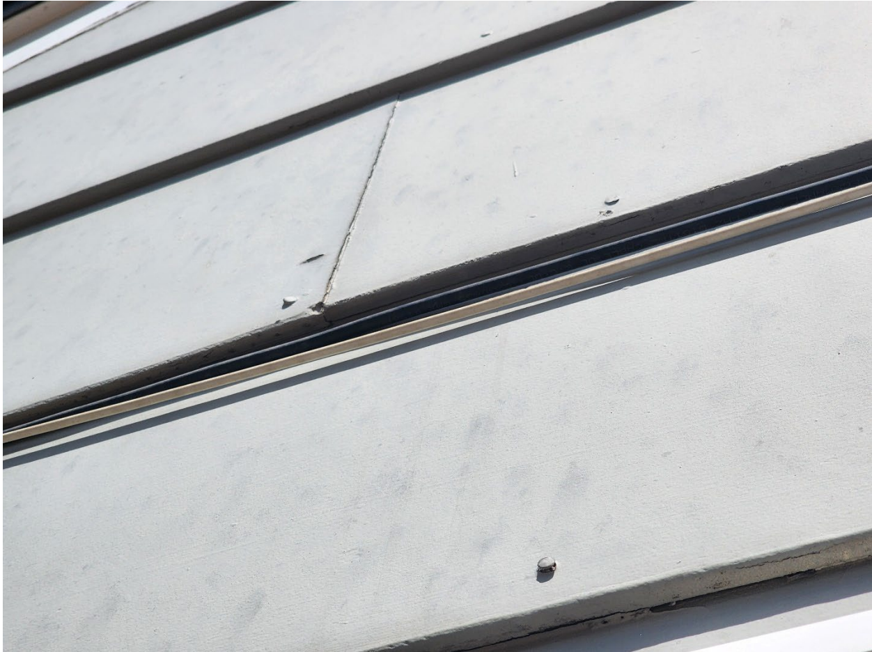
Figure 33: West Wall of 1957 Ranch in Colorado, Nails Visibly Working Their Way Out of Fiber Cement Siding (Lord, 2023)
