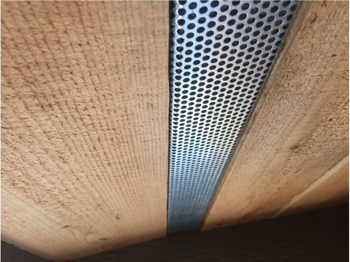
Figure 42: Vulcan Vent Soffit Vent, Accessed May 22, 2023
