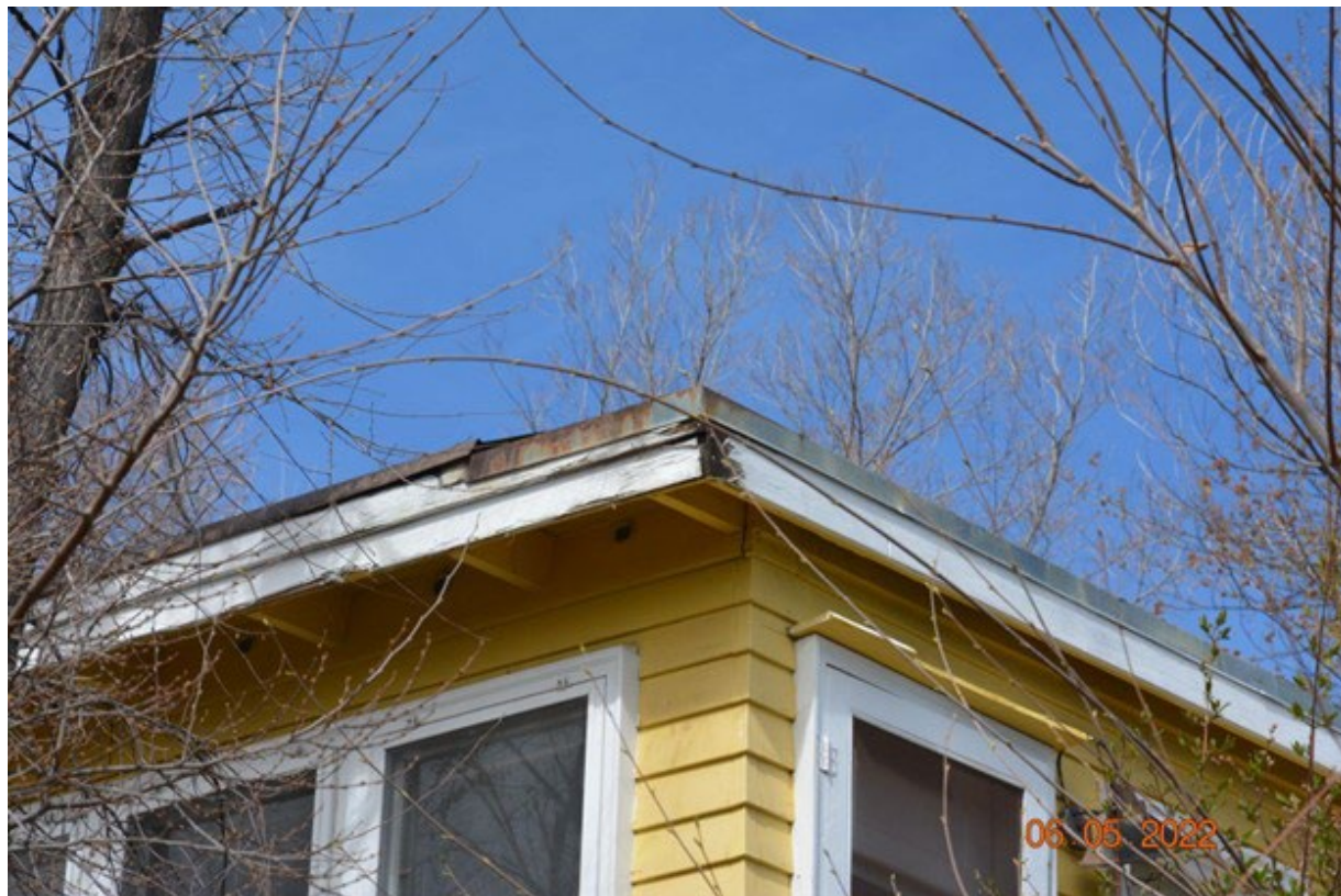
Figure 8: Deteriorated fascia board that provides an entry for wind-blown embers can result in an ignition on the interior of the structure.
