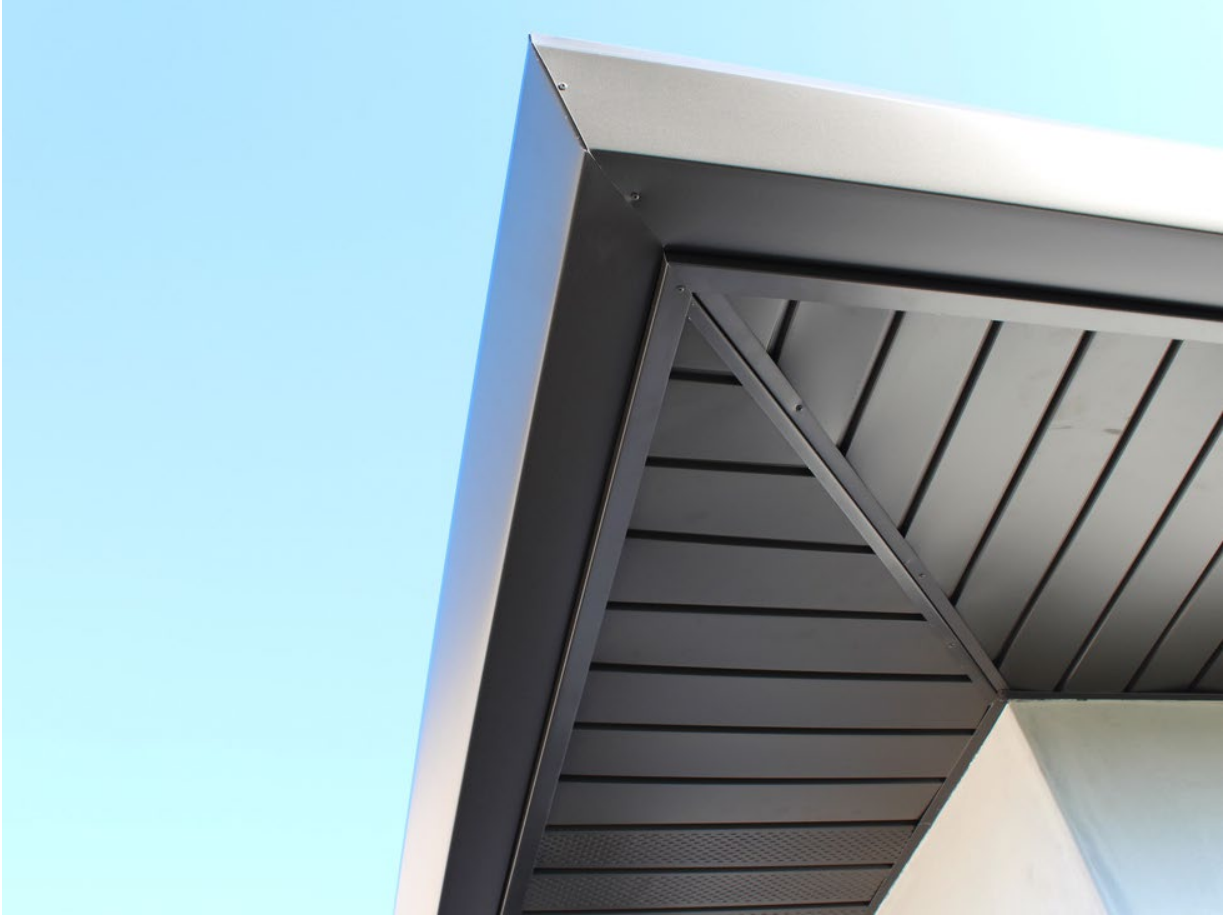
Figure 19: A Plus Gutter Systems of Los Angeles and Orange County, Photo of soffit and fascia retrofitting with sheet metal, Accessed May 17, 2023
