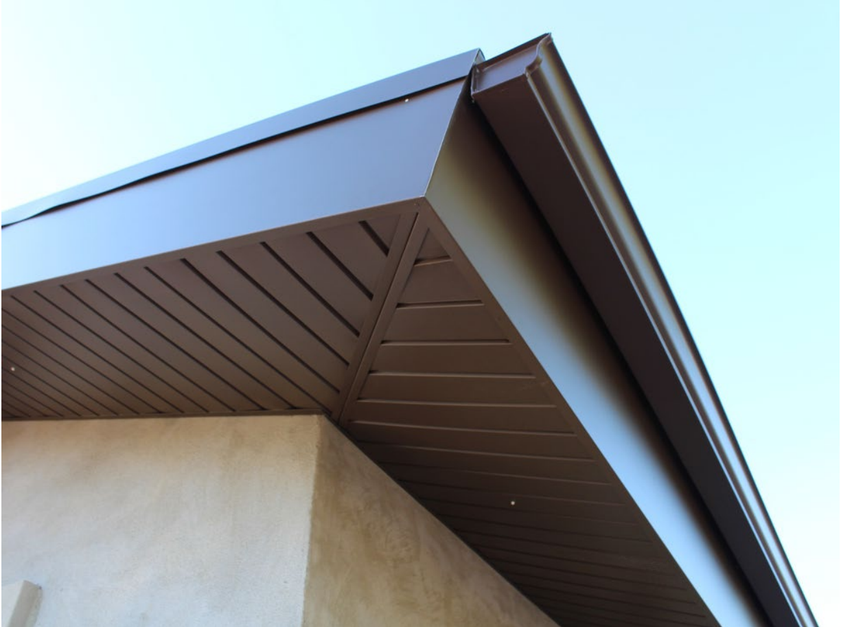
Figure 20: A Plus Gutter Systems of Los Angeles and Orange County, Photo of soffit and fascia retrofitting with sheet metal, Accessed May 17, 2023
