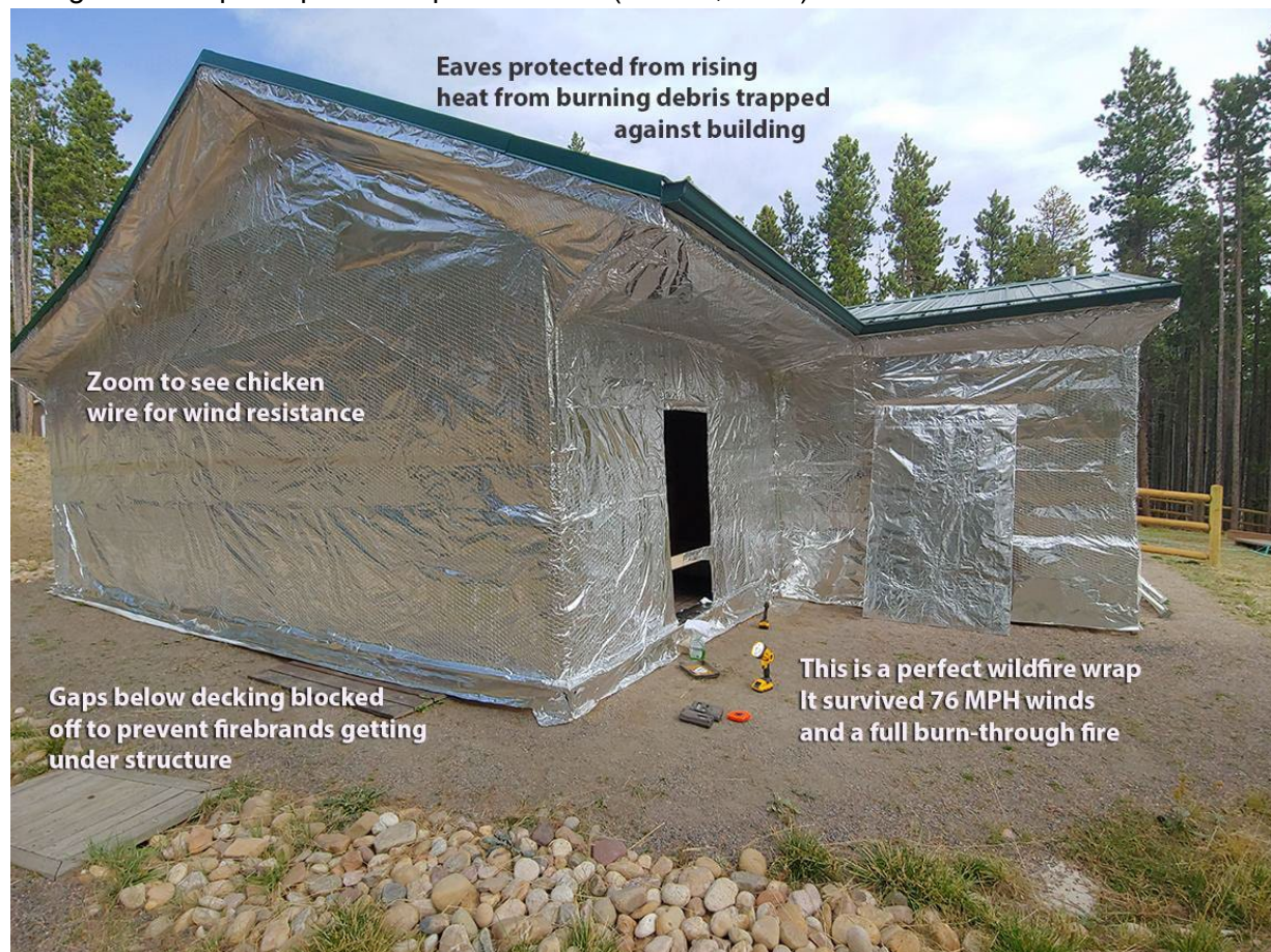
Figure 10: Firezat installation with chicken wire and staples. Building has an existing metal roof eliminating the need to wrap the roof. Image credit: firezat.com, accessed March 21, 2023
