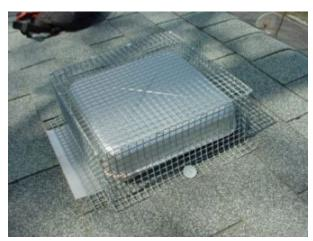
Figure 37: Roof Vent with Retrofitted Wire Mesh Cover (Roof Vent Screens Installation, 2023)
