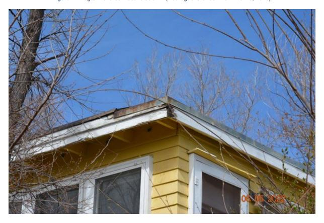
Figure 8: Deteriorated fascia board that provides an entry for wind-blown embers can result in an ignition on the interior of the structure.
