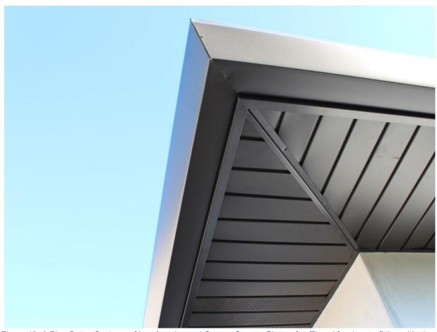
Figure 19: A Plus Gutter Systems of Los Angeles and Orange County, Photo of soffit and fascia retrofitting with sheet metal, Accessed May 17, 2023
