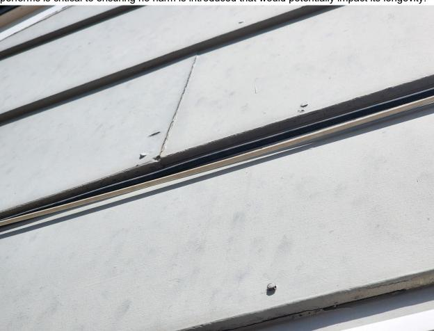
Figure 34: West Wall of 1957 Ranch in Colorado, Nails Visibly Working Their Way Out of Fiber Cement Siding (Lord, 2023)
