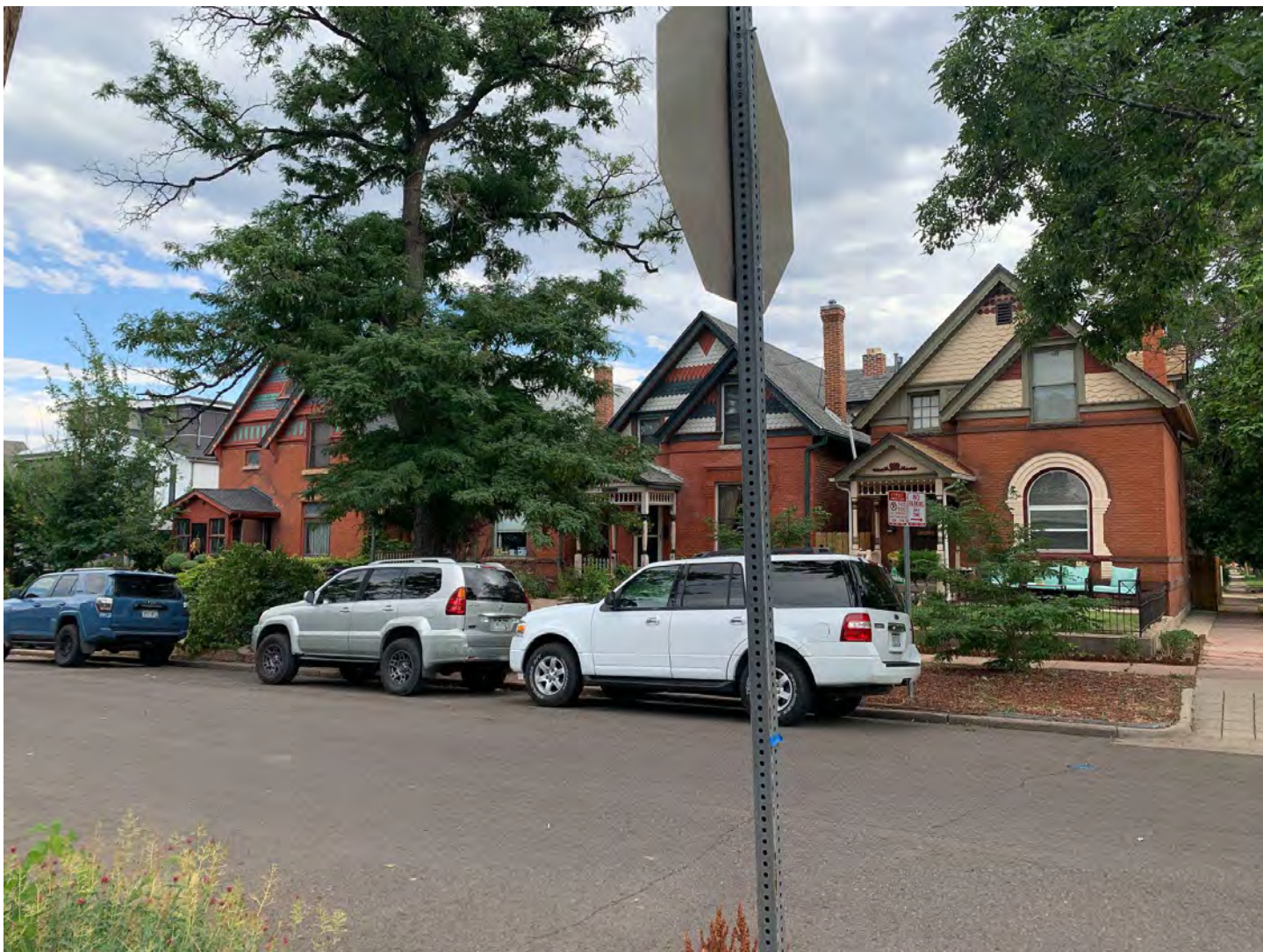
65. View from corner of 34th Ave. and Wyandot St.. Right to left- 2258, 2254, 2250, 2246 W. 34th Avenue. Photo taken July 22, 2022.
