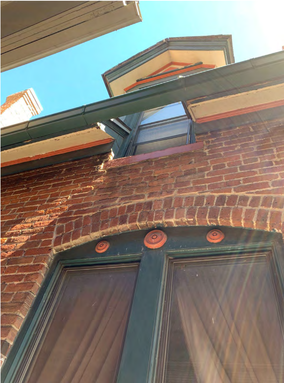
9. Photo of the first floor west-facing sitting room window with decorative molding, and brick semi-arch. Above, is the second floor west-facing dormer window with decorative trim and molding. Photo taken September 19, 2022.
