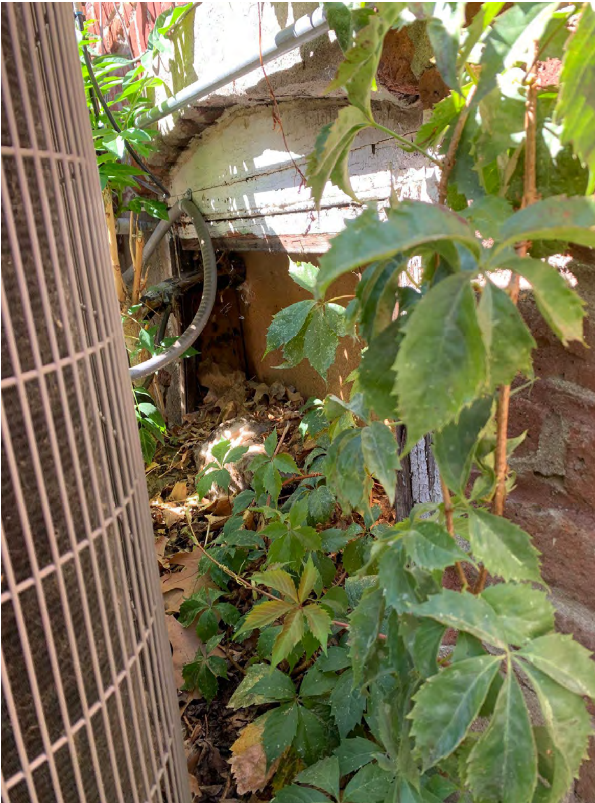
13. South-facing cellar window covered with interior wood board. Photo taken September 19, 2022.
