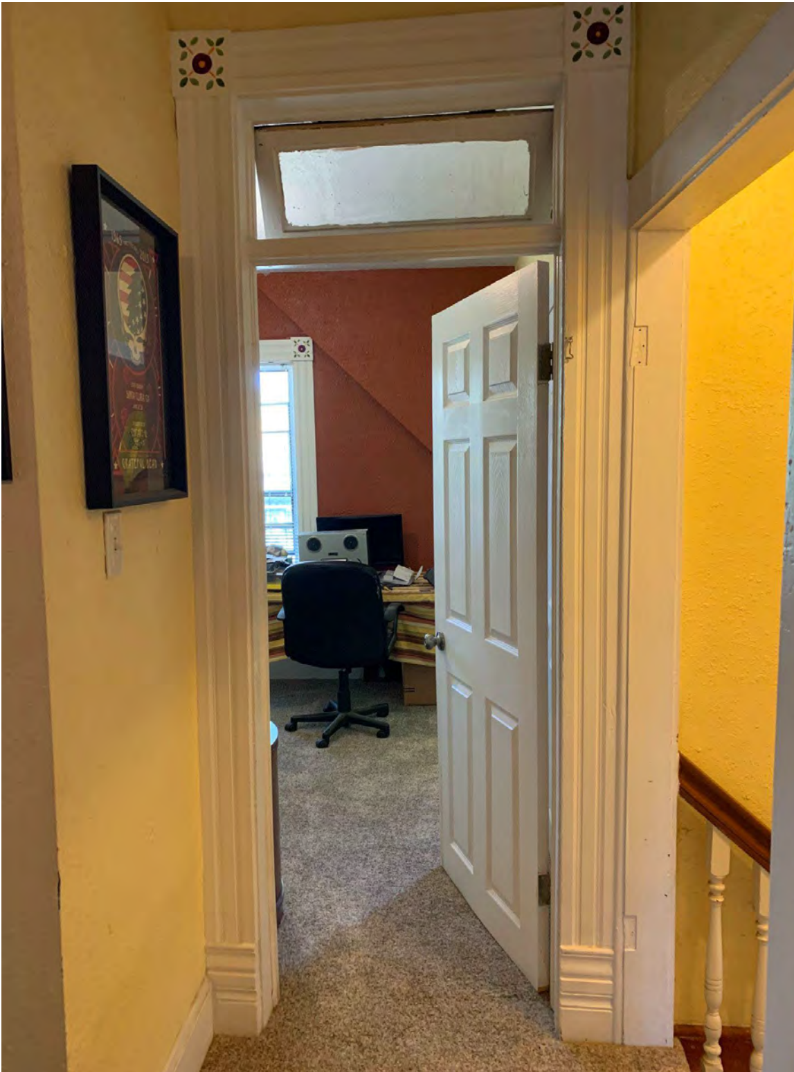
45. View from sitting room toward guest bedroom doorway with glass-paned transom. Note the spaces where hinge plates used to support a locking door at the top of the stairs. Photo taken September 26, 2022.
