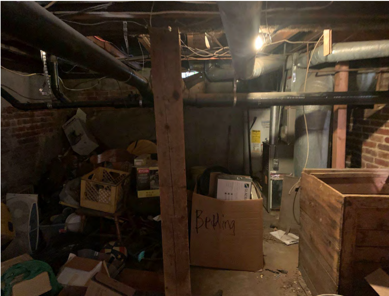
35. Cellar view from the bottom of the stairwell. Photo taken September 26, 2022.
