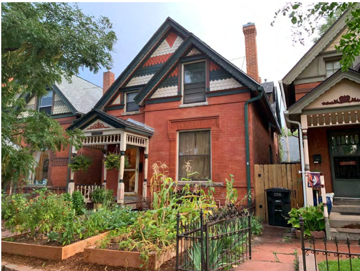
1. North (front) facade, camera facing southeast. Note the scalloped and shaped shingles, turned spindles, multiple gables, and decorative entry porch. Photo taken September 14, 2022.
