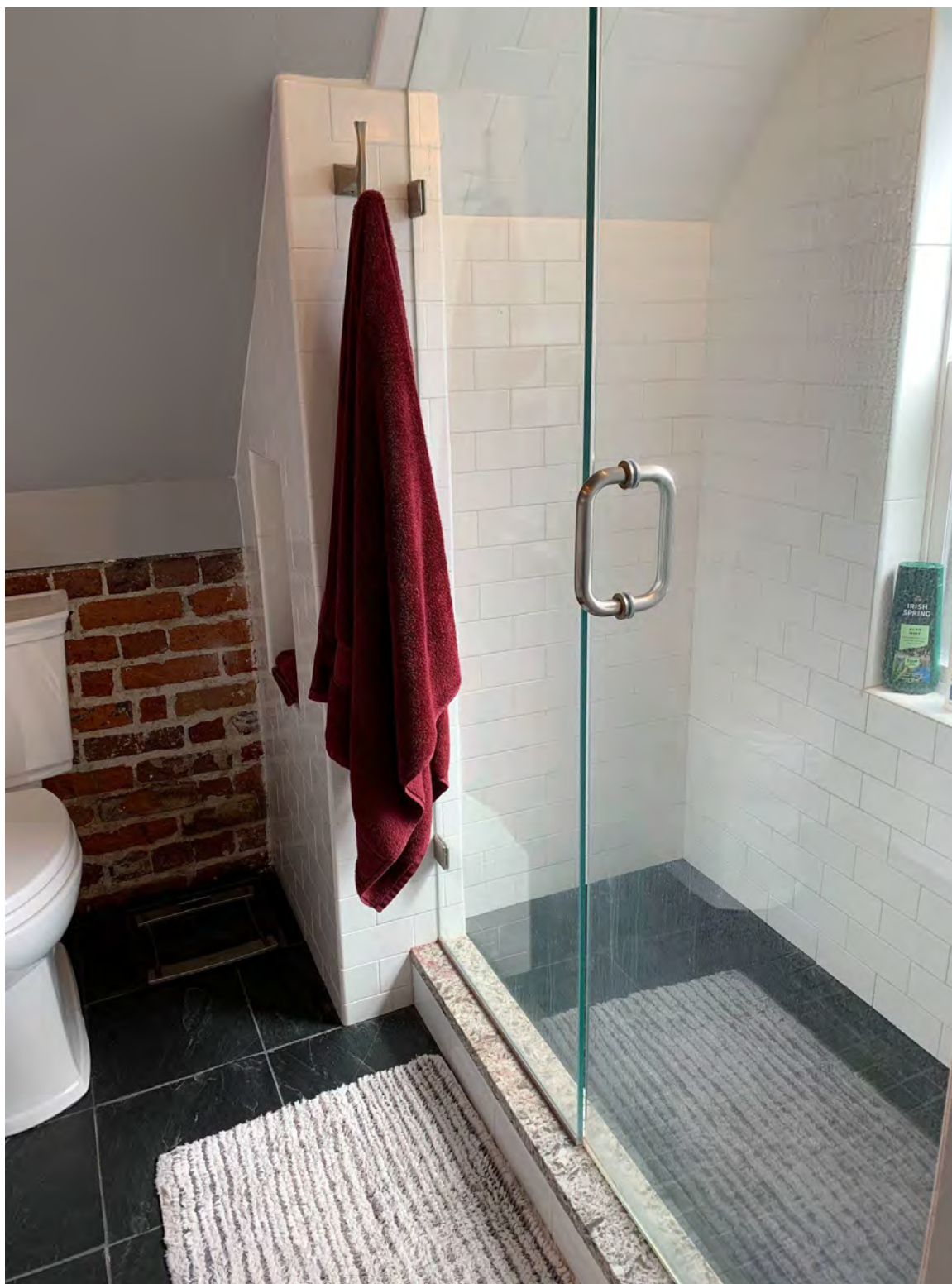
55. Main bathroom renovated in ca. 2019 with west-facing privacy window to the right. Photo taken September 14, 2022.
