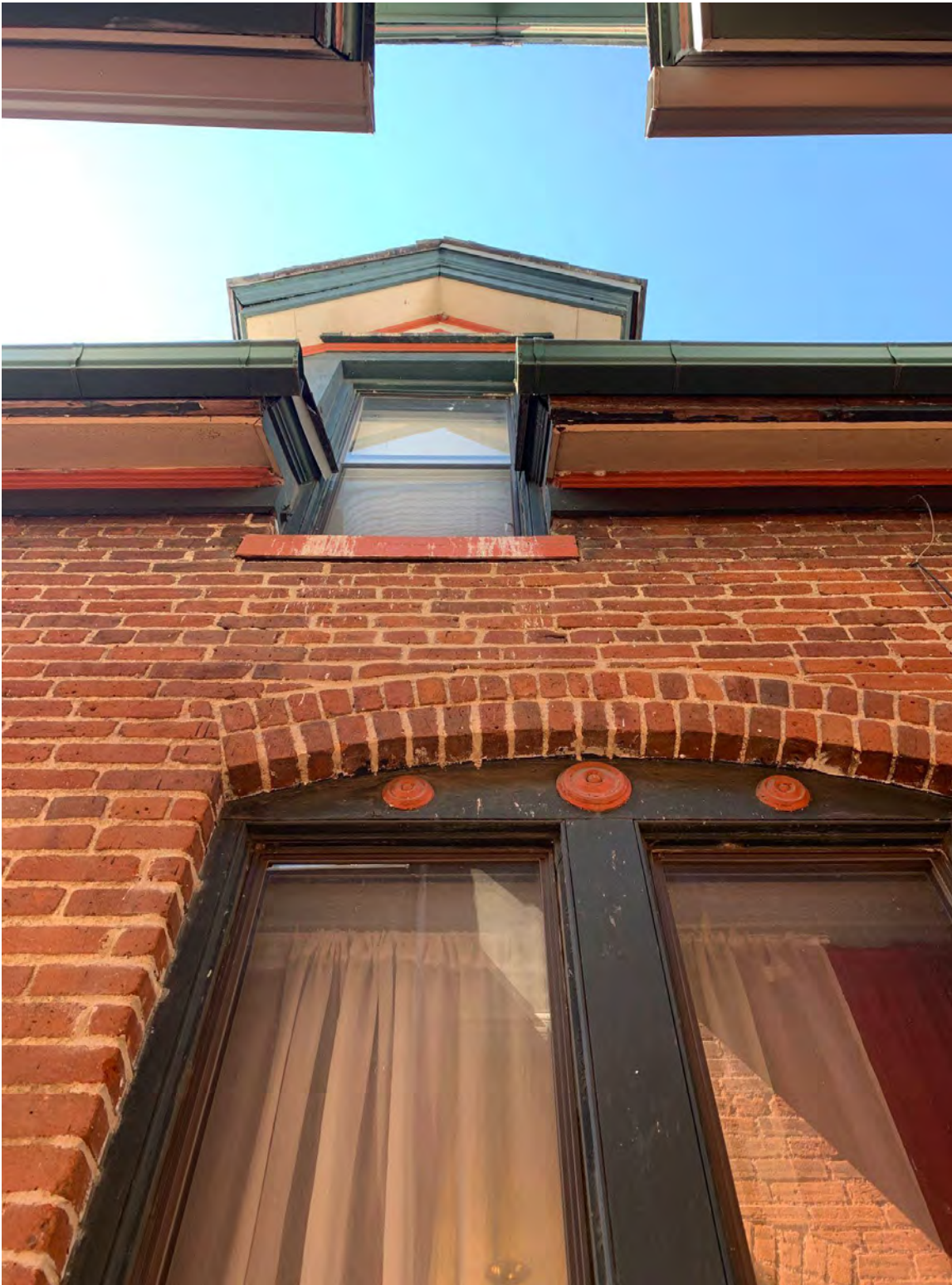
6. Photo of the first floor east-facing dining room window with decorative molding, and brick semi-arch. Above, is the second floor east-facing dormer window with decorative trim and molding. Photo taken September 26, 2022.
