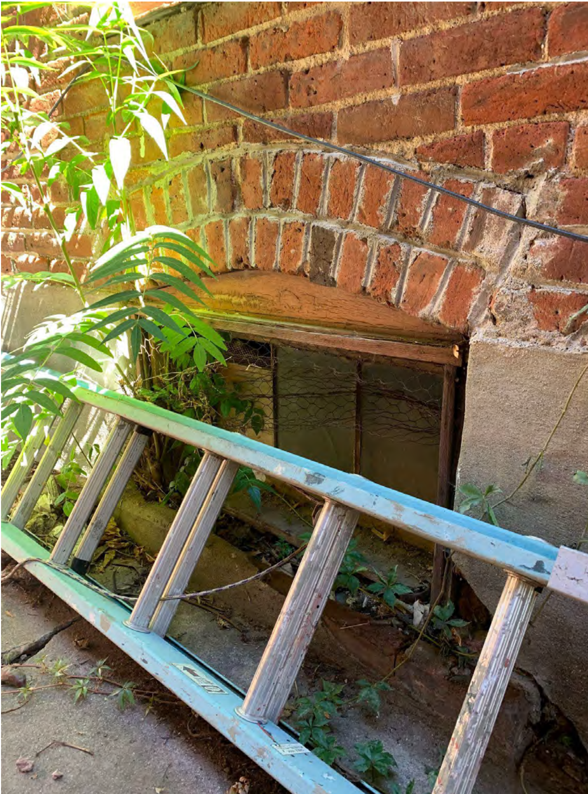
10. Original west-facing cellar window. Photo taken September 19, 2022.
