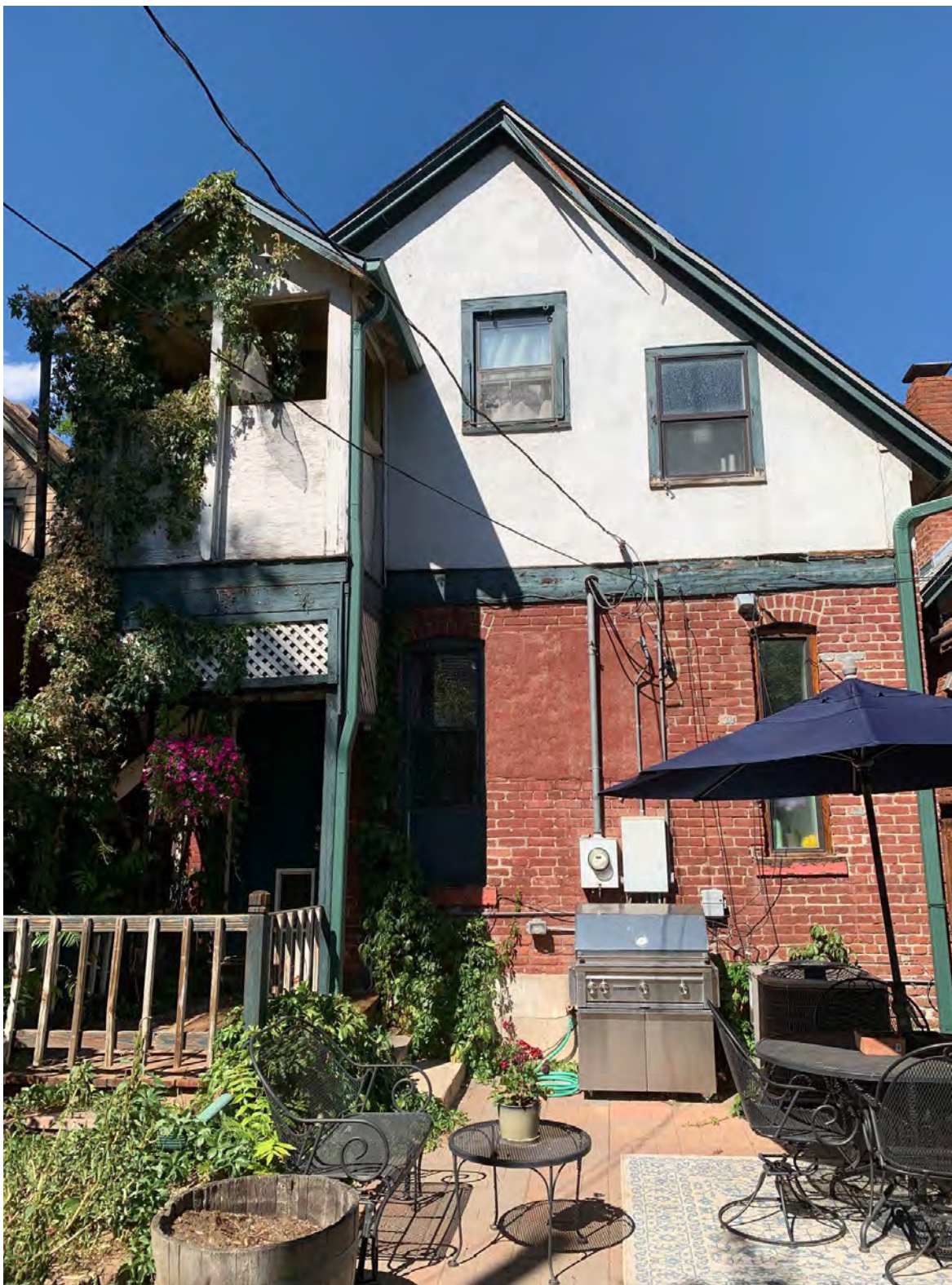
11. South-facing facade (backyard) with red brick first floor and kitchen entry porch and railing formed by the above main bedroom balcony. Note the second floor plaster/stucco facade of the main bedroom addition in the mid- to late-1930s. Photo taken September 19, 2022.
