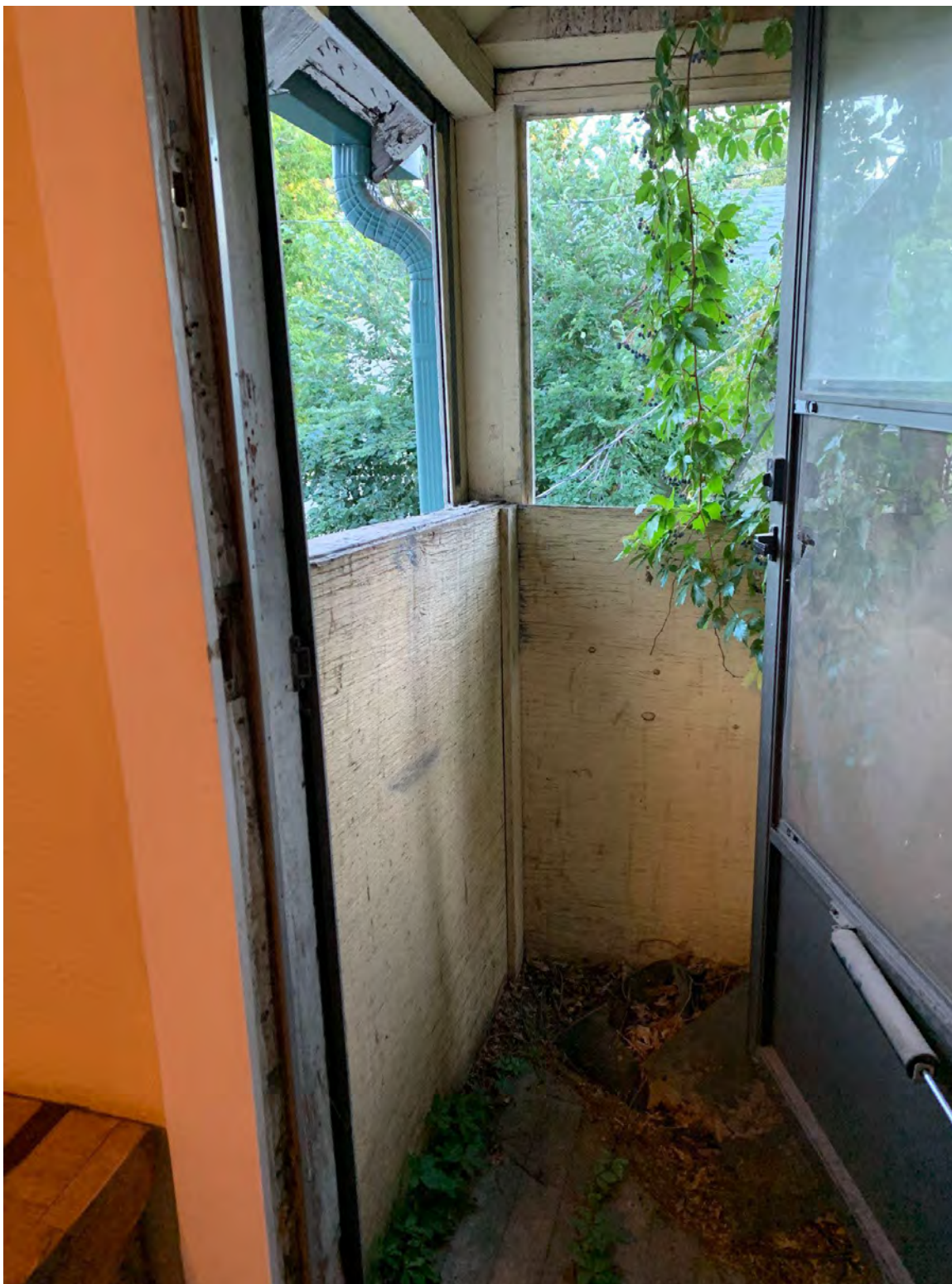
57. View of the covered 4' x 6' balcony porch from the main bedroom. Note the once screened-in windows. The balcony is currently unsafe for use. Photo taken September 26, 2022.
