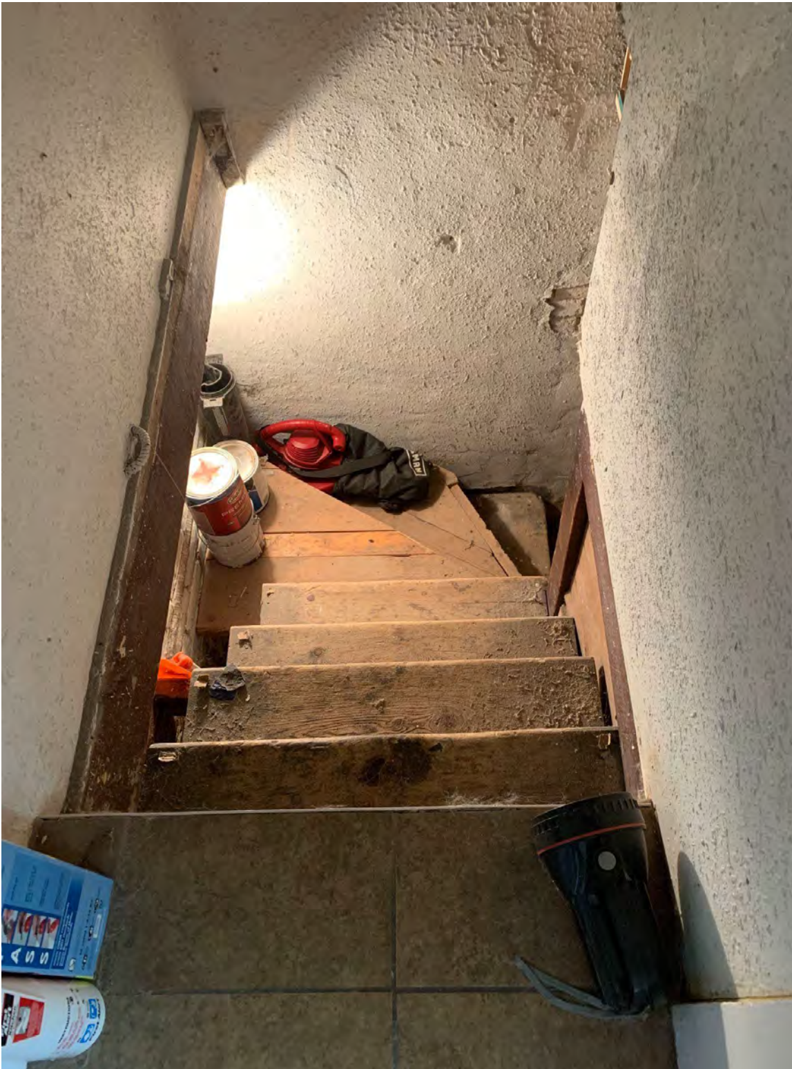
34. Stairwell leading into the cellar from the kitchen. Photo taken September 26, 2022.
