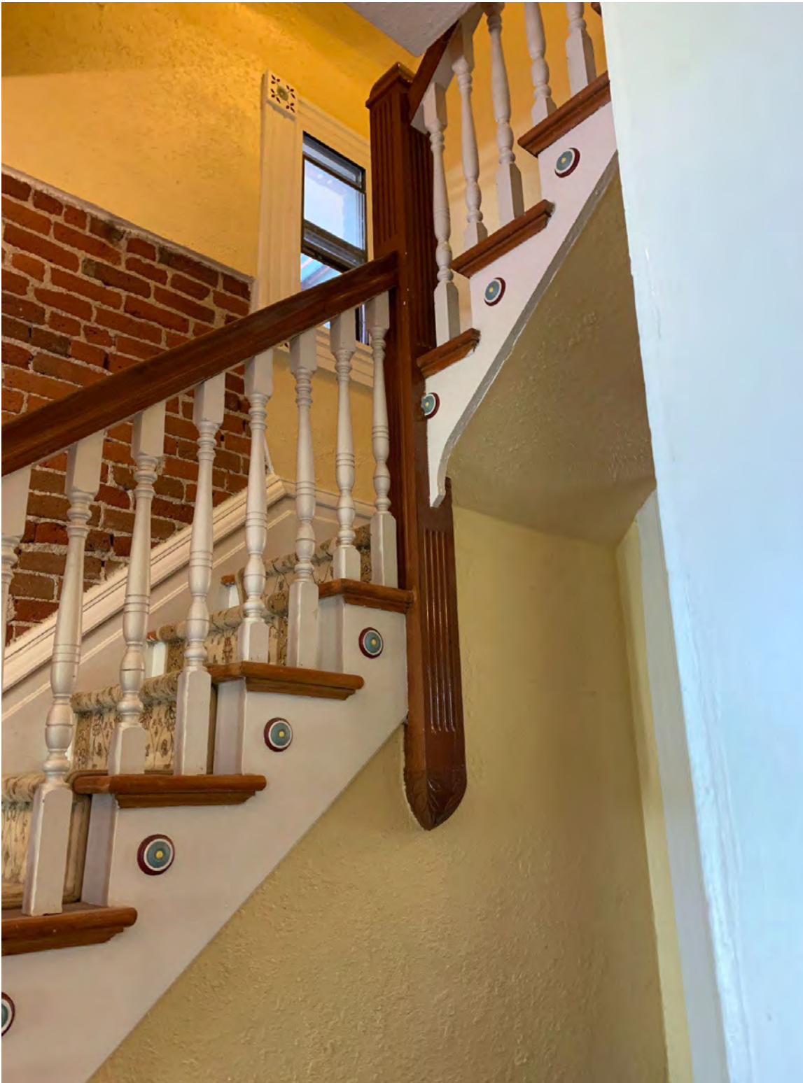
40. Stairwell detail and handcrafted landing newel. Photo taken September 26, 2022.
