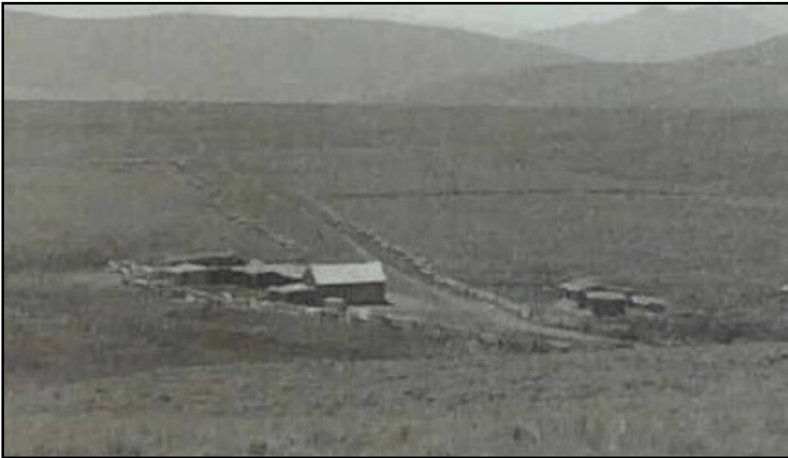
Figure 2. Same photo as Figure 4, cropped to emphasize the buildings. Note wagon road (Feature 10) between the Selak barn (Feature 2) on eastern side, and the general store (Feature 4) and other buildings on the western side. Today, that road has become an eroded drainage that bisects the site.
