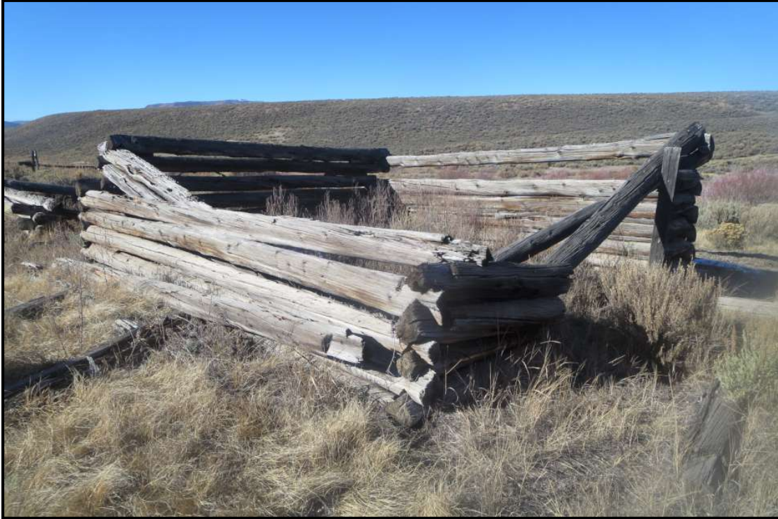
Photograph 10: Feature 4 with Feature 3 (background, L)
