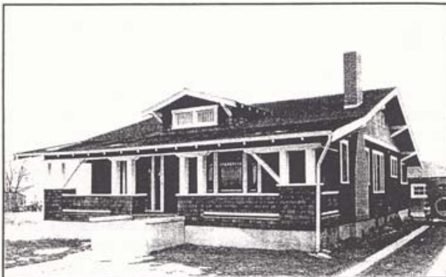
Figure 14. This Craftsman/Bungalow style residence at 5626 South Crocker Street was erected by Dan S. Reid Construction Company in 1921 and is notable for its shingled walls and broad porch. SOURCE: Littleton Historical Museum, photograph number 1990.
