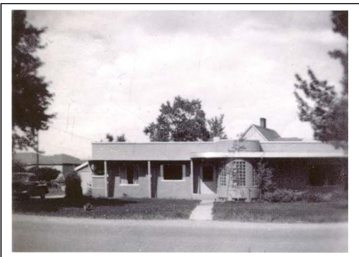
Photo H3- House in 1954. Interior yet to be completed.
