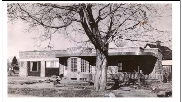
Photo H2- South elevation, brick & block structure waiting for stucco. Window in brick section yet to be placed. Date Unknown.
