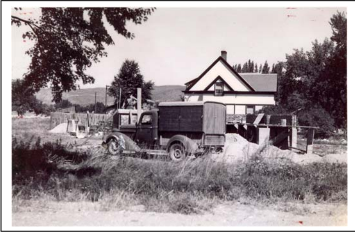
Photo H1- South facade, brick structure seen at west end. Date unknown.
