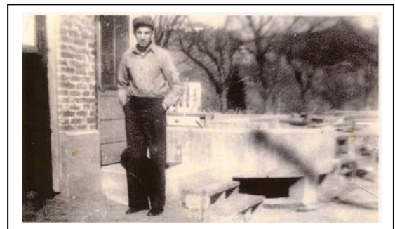
Photo H4- Elwood Heister at south secondary entry- basement started. Date unknown, probably 1942-43.
