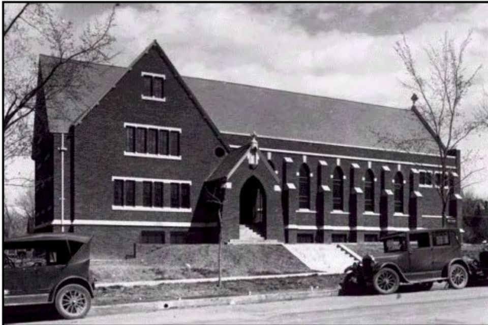
West elevation of the University Park Methodist Episcopal Church about 1928 Photographer: Unknown. Source: Western History/Genealogy Department, Denver Public Library
