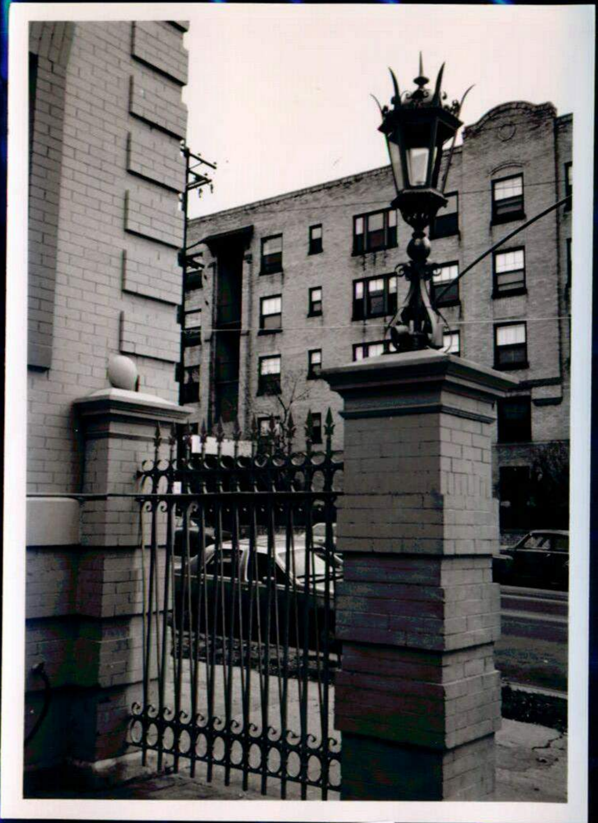
1985 view South Courtyard entry
