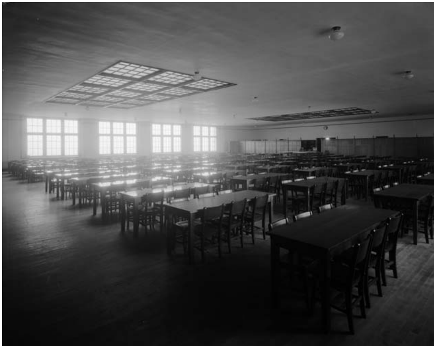
Figure 9. This circa 1925 view shows the original lunchroom that was converted to science classrooms in the 1972-74 school remodeling and expansion.
