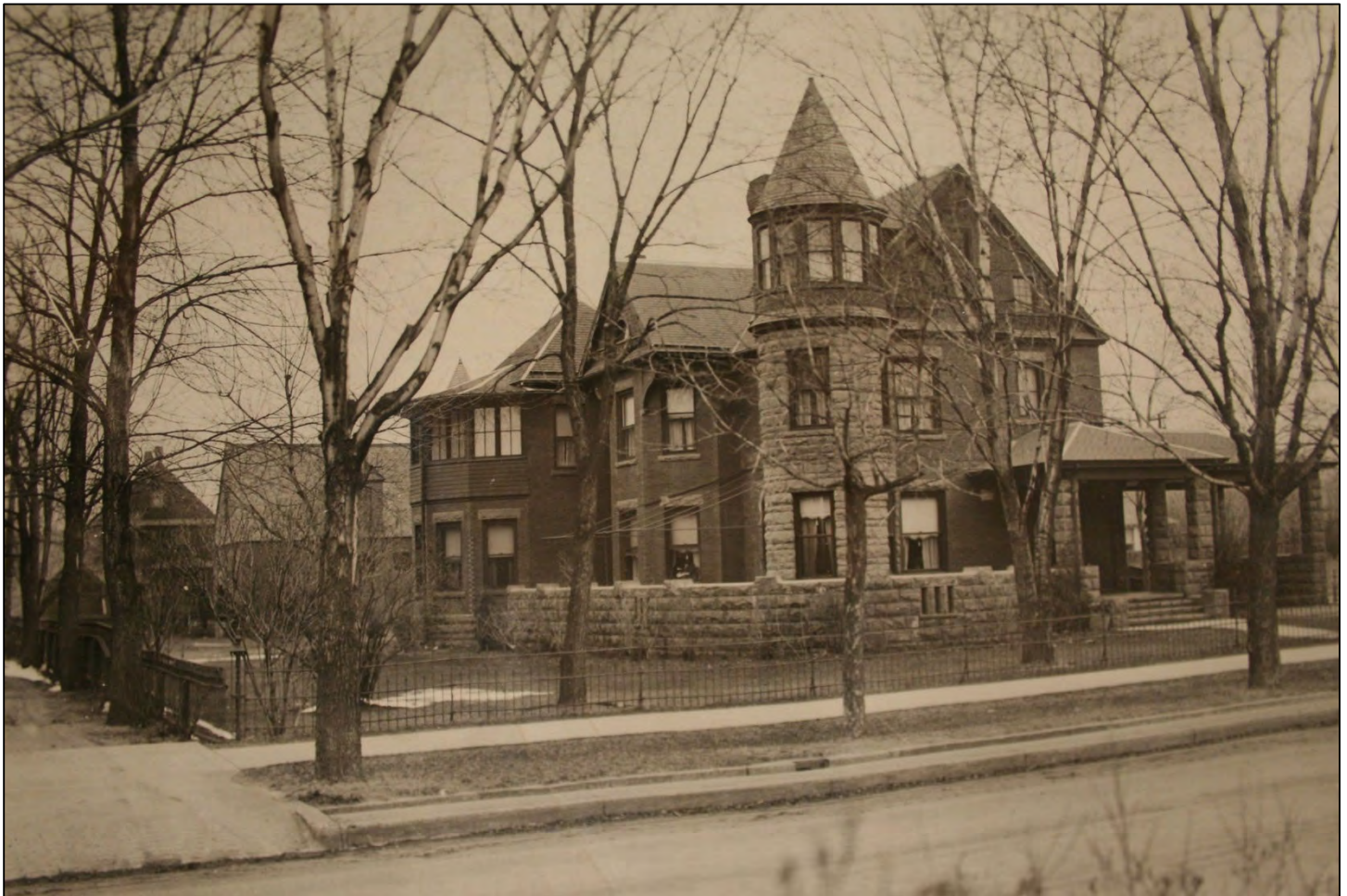
Figure 4. This 1920s or 1930s view northwest shows the house after the reconfiguration of the porch and construction of the porte cochère on the north and the semi-decagonal tower at the southwest. The carriage house is visible at the rear immediately to the left of the house. Courtesy of Colorado College Special Collections, Morreale House, ca. 1920s, Colorado College Photo Files, Buildings.
