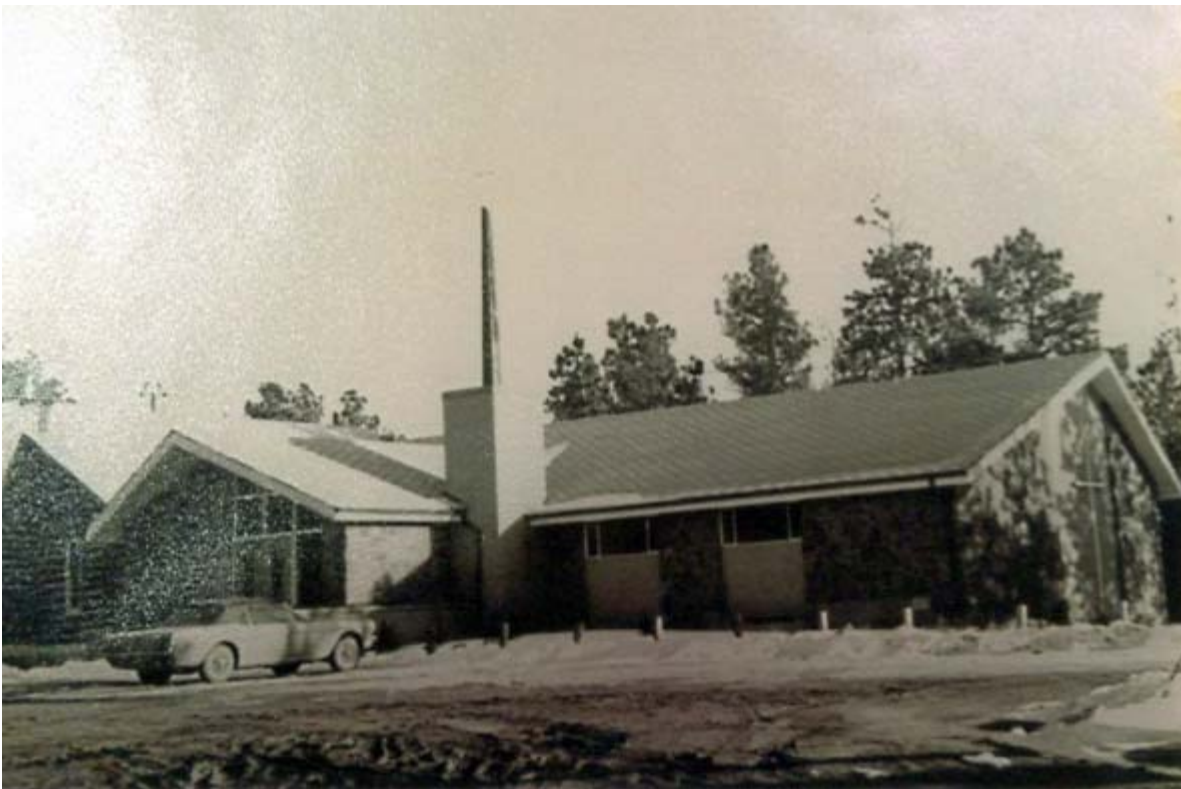
Historic Photo 6 - Stone Church Building, 1962, North and West Sides
