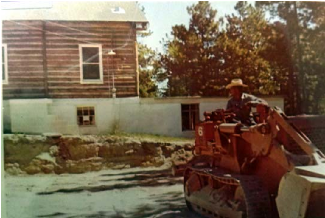
Historic Photo 1- Log Building, West Side, showing 1953 Basement Addition
