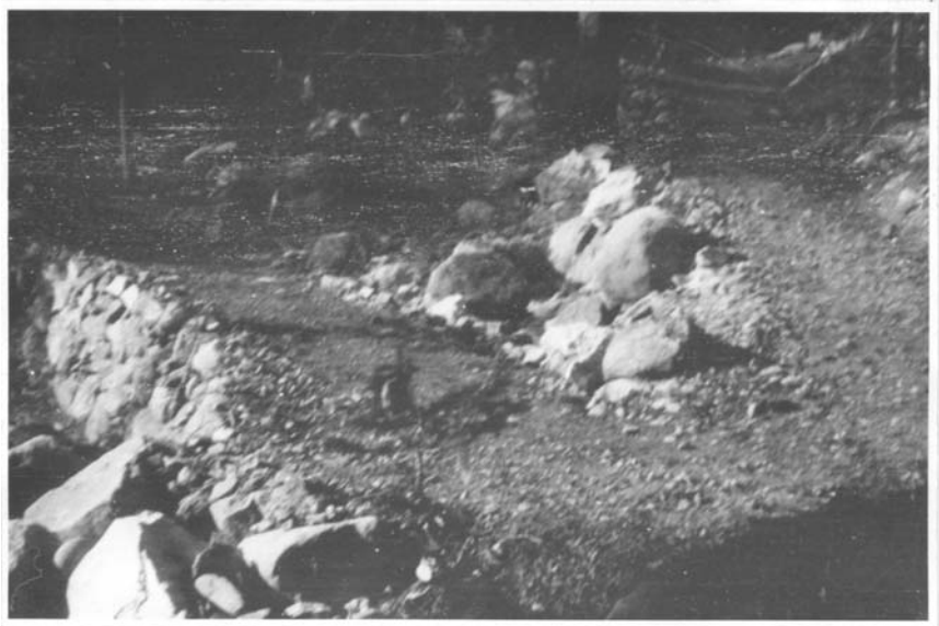
Switch Back No. 1, 1930, (Station 56 plus 42)
