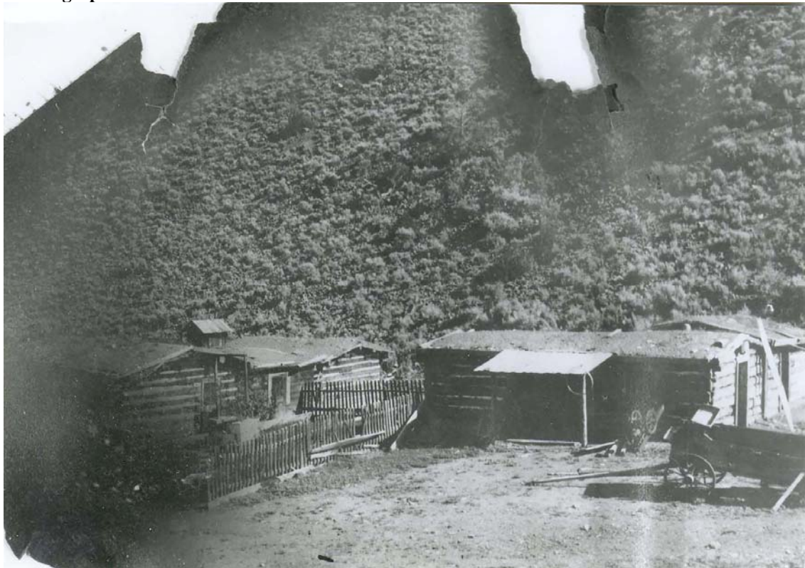
H001: An early view of the complex of log cabins at Johnson Stage Station, ca. 1889. Facing east, Johnson Cabin and the Saloon are to the left and Guest Cabin to the right
