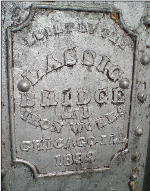
Figure 3: Stamp showing manufacturer and date of construction, Bridge #2
