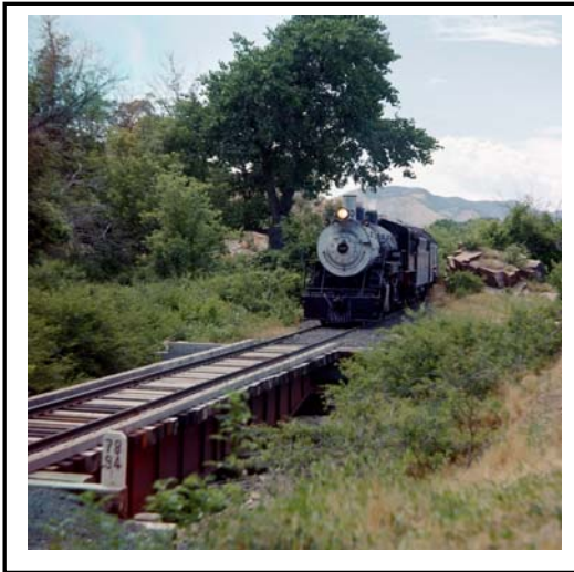
Figure 4: Locomotive crossing Bridge #2, heading east. Circa 1955.
