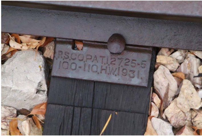
Figure 2: Tie plate, tie, rail and ballast
